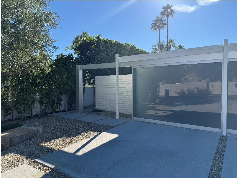
Garage door detail.
