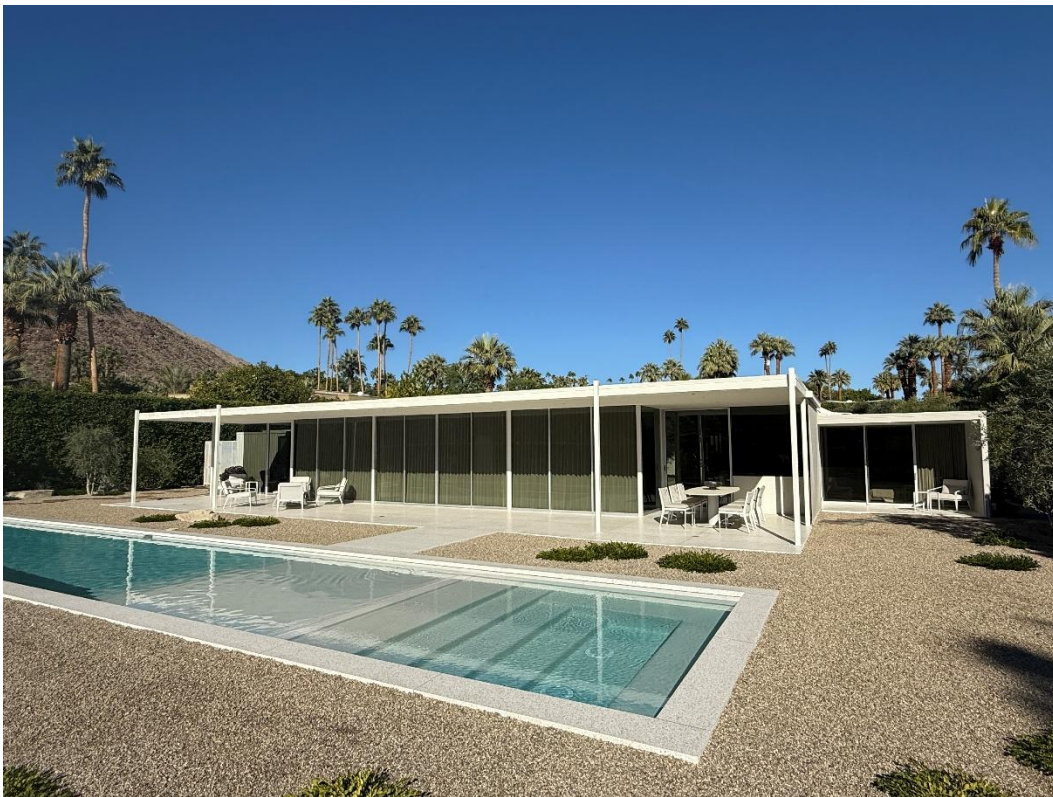
The deep overhang at the rear of the house with Cody's signature impossibly thin steel posts and beam, shading the rear wall of the house, which is entirely floor-to-ceiling glass.
