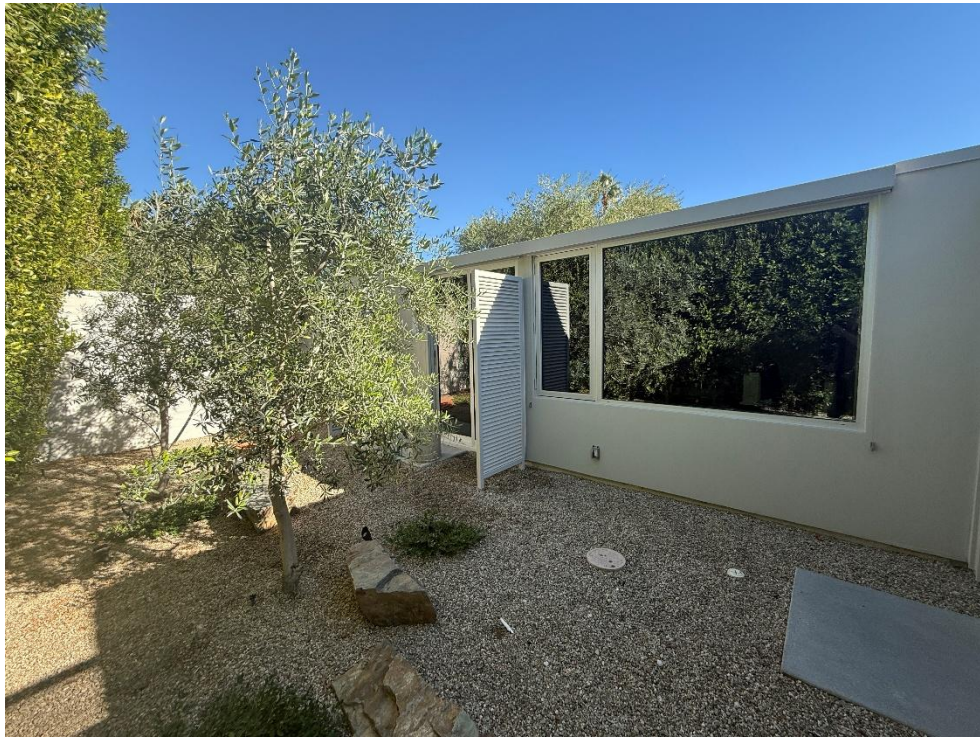
The small private patios of the bedroom wing on the west elevation.
