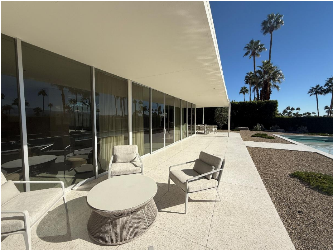
The rear terrazzo deck with deep overhang above.
