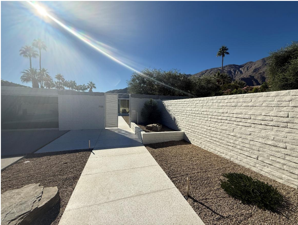
Views of front garden showing white-painted slumpstone walls and minimalist landscape. Note slumpstone planter to right of front gate.
