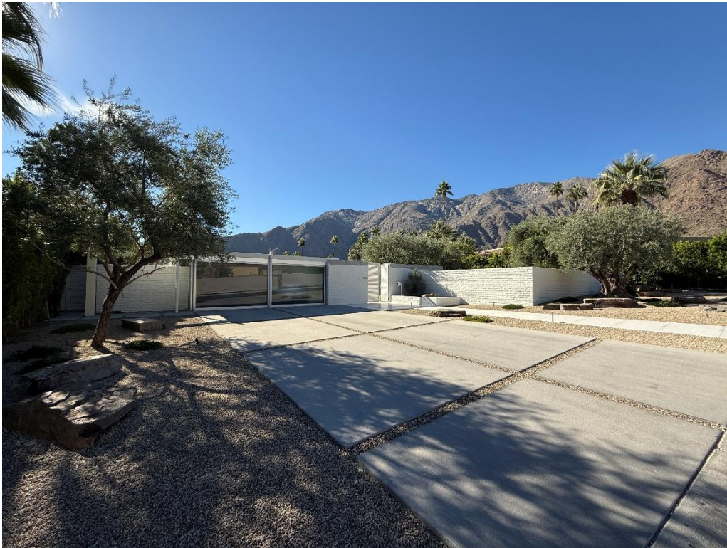
Looking southwest towards garage and driveway, and path leading to front gate, with slumpstone wall.
