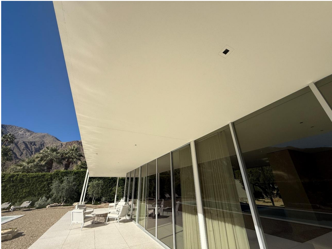
More details: original aluminum hardware on the original anodized aluminum sliding glass doors; walls of floor-to-ceiling sliding glass doors and fixed panels of glass.
