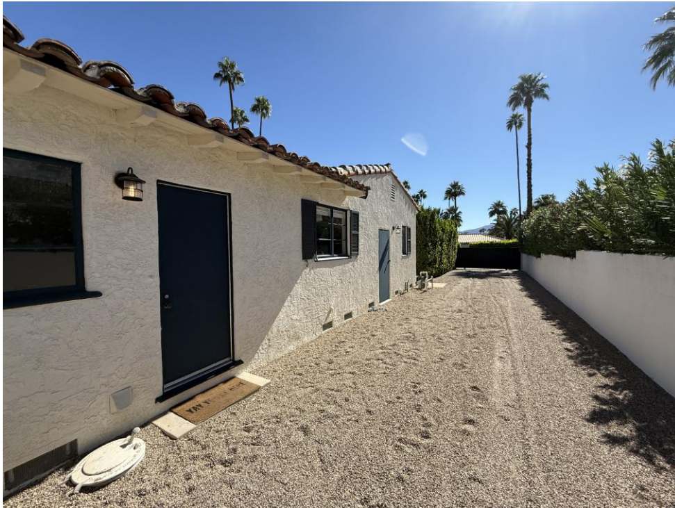
Closeup view of steel casement windows, showing the hardware for the shutters, which are missing, top. The bottom photo shows the service wing of the house and the driveway. Note the original trash compartment sunken into the ground at bottom left.
