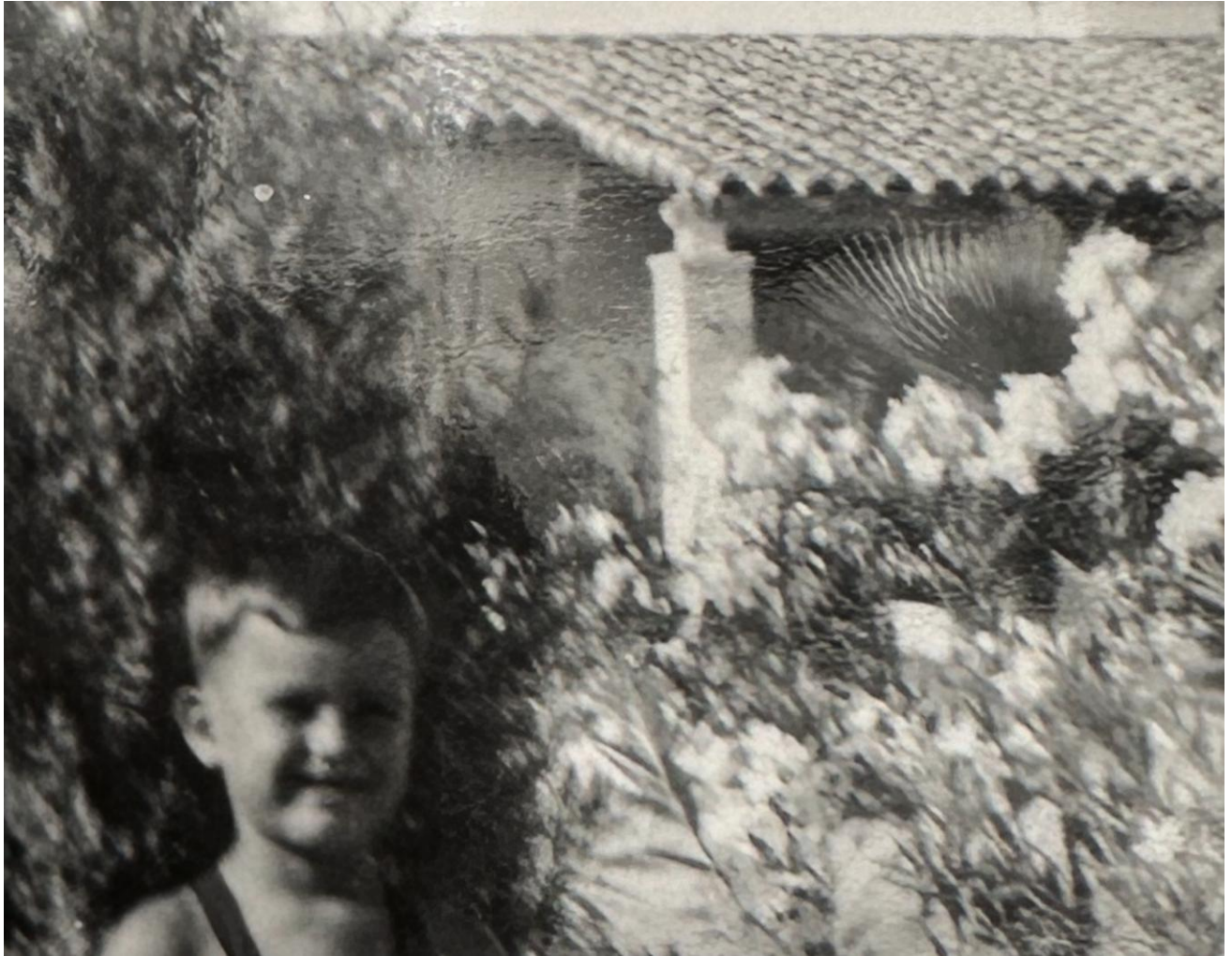
In this detail from an early photograph, the stacked Mission tile finials atop the brick columns are visible, painted a light color.
