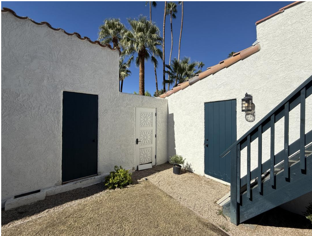
Views of the rear patio. Note rebuilt stairs leading to roof deck.
