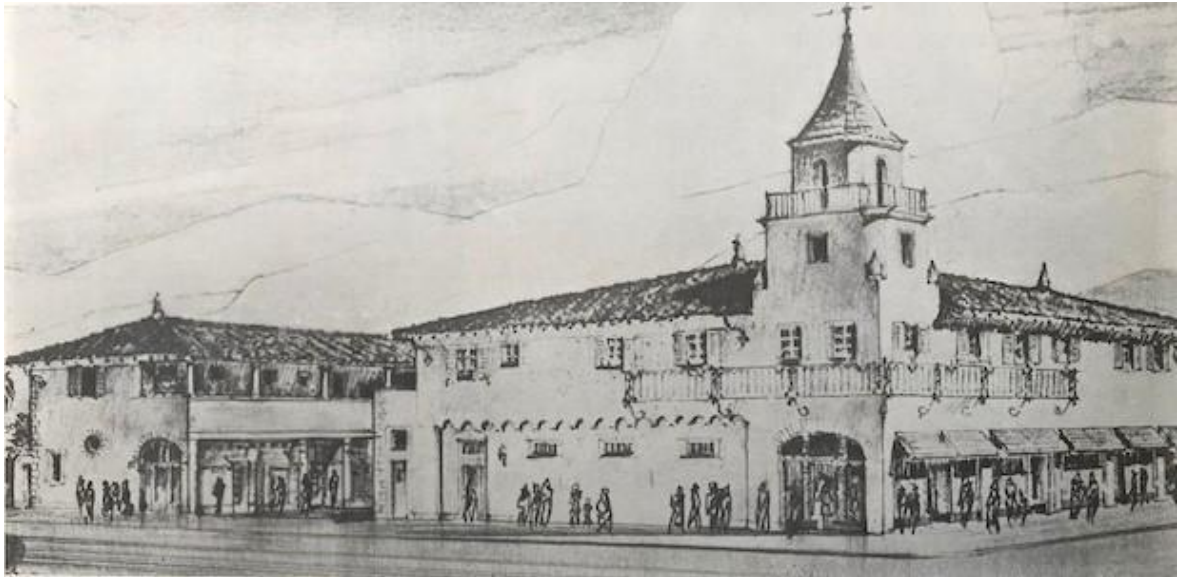
Pacific Building, 1937. Brewster & Benedict, architects
