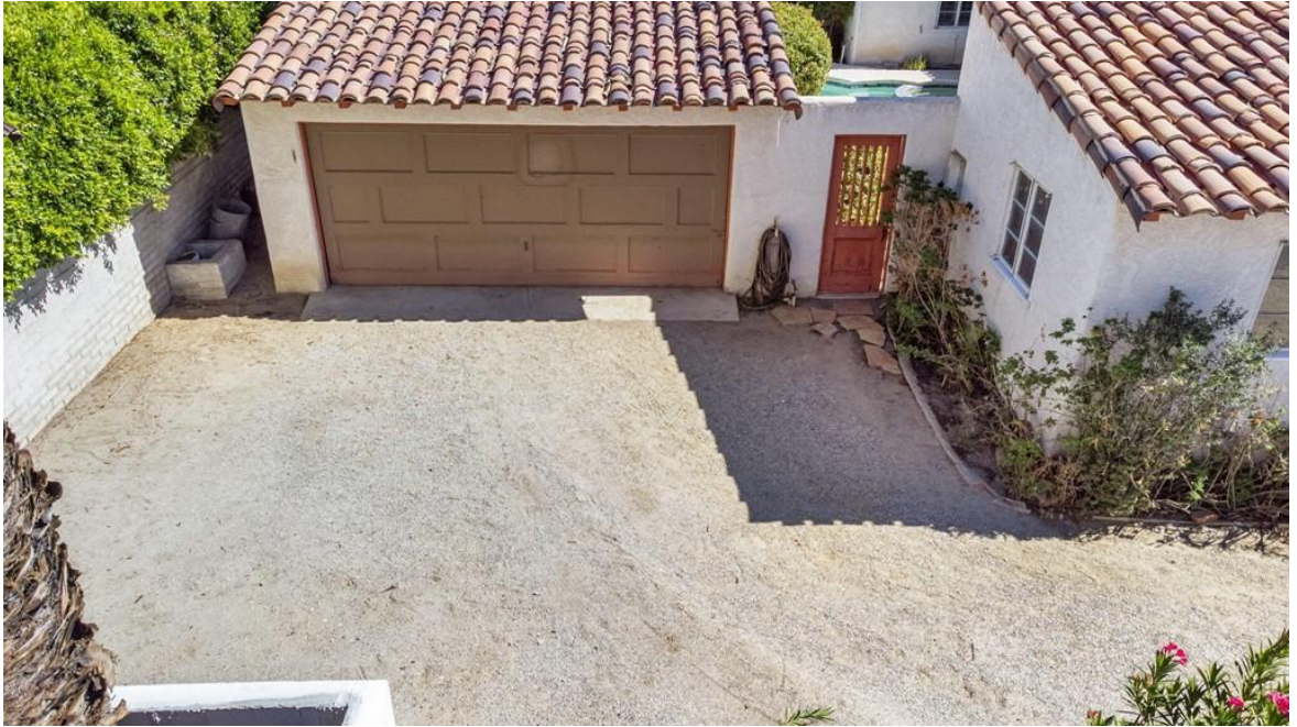
The detached garage and driveway.
