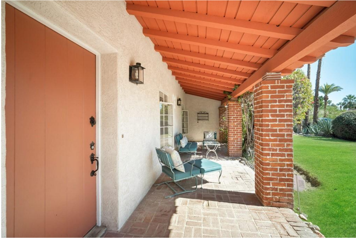
In this photograph from the 2021 sale, the original configuration of the brick columns with stacked Mission tile finials is visible. They were later modified to extend the brickwork to the top.
