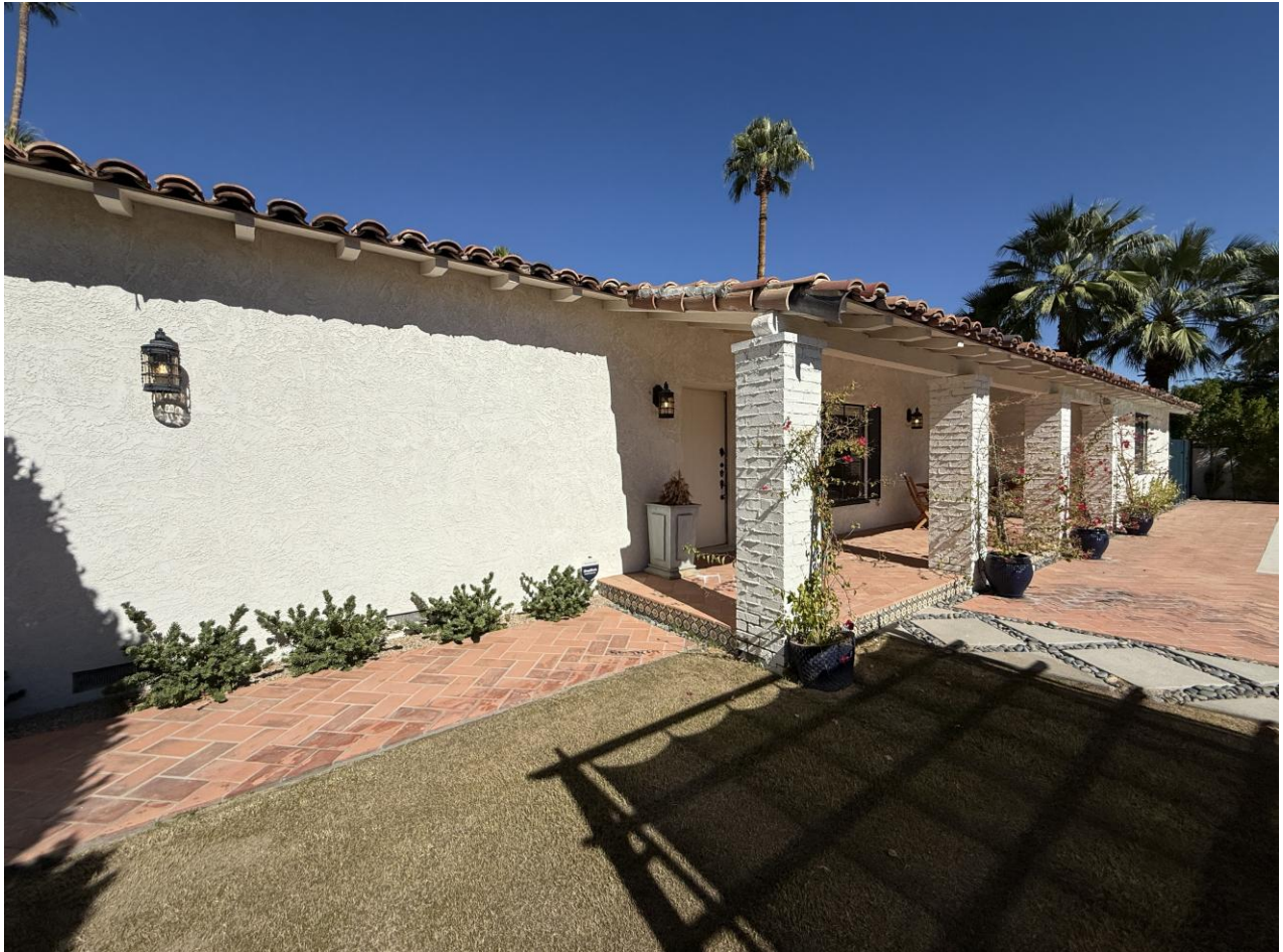
View of primary façade, 2025.
