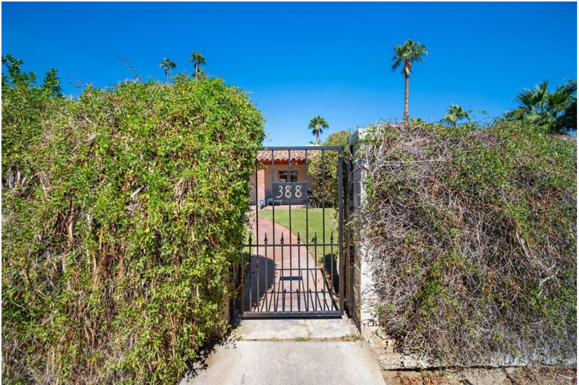
A wrought iron gate has replaced the original wooden gate.
