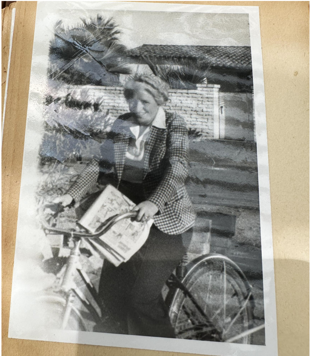
This later photograph from roughly the same location shows the brick wall with weeping mortar joints has been built, with wood gate for pedestrian access.
