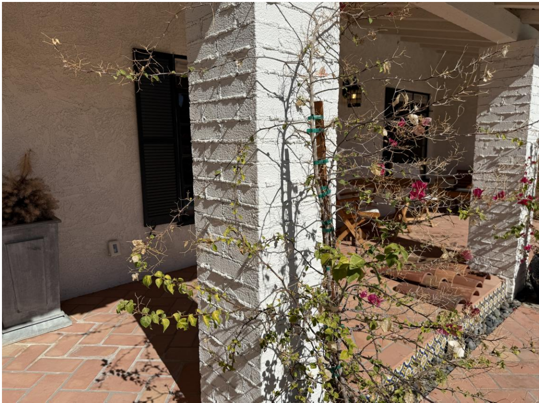
Views of primary façade and brick column detail.
