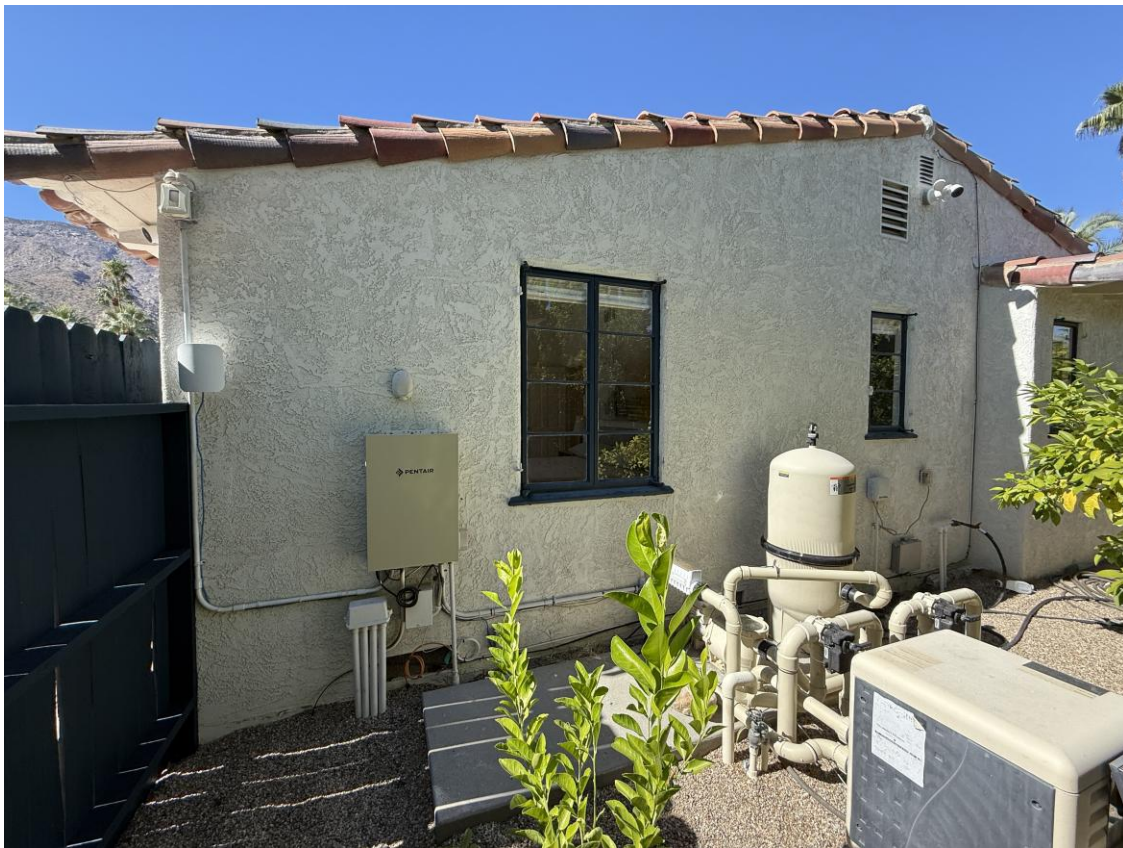
Views of the bedroom wing to the east of the structure.
