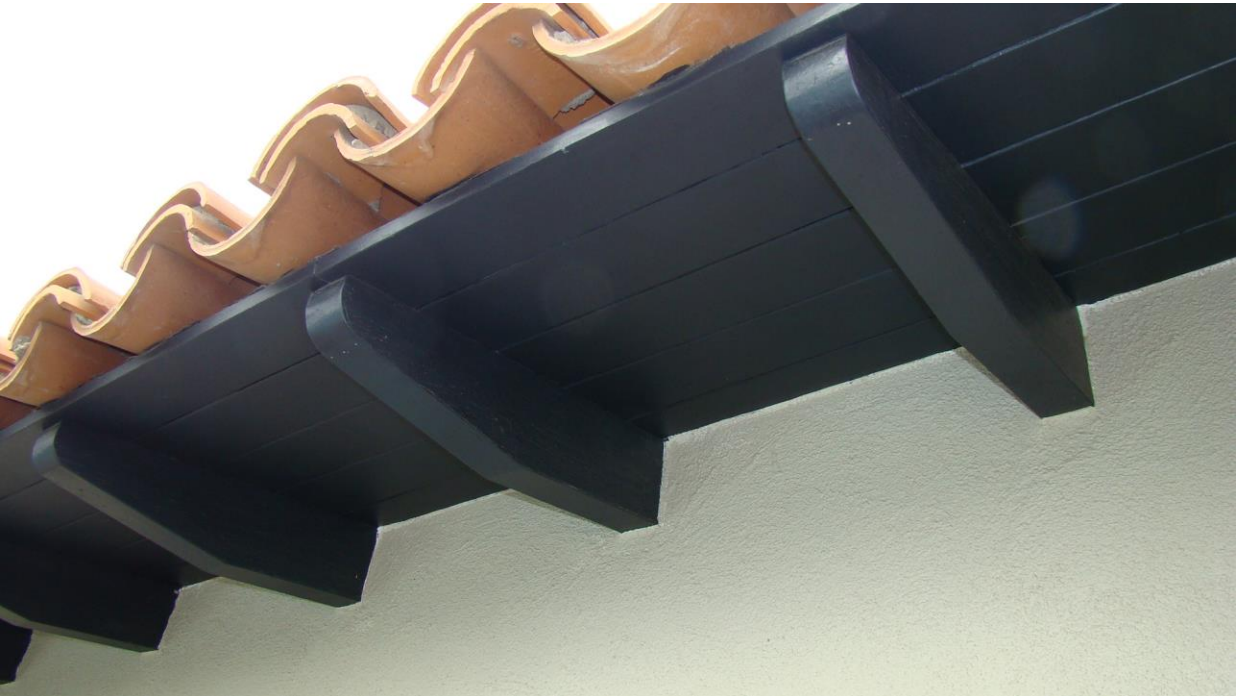
3"x6" Tapering Wood Roof Rafters which feature Rounded Tips
