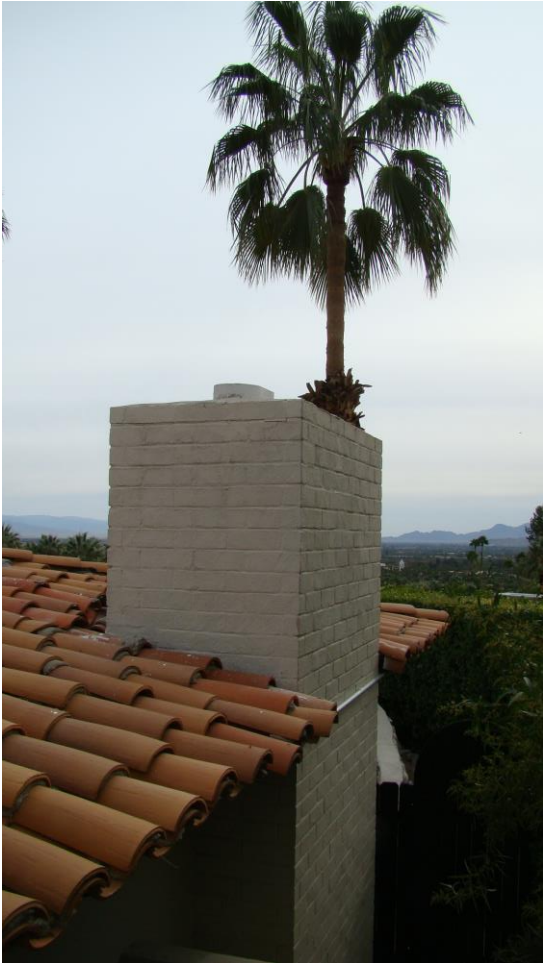
Concrete Block Fireplace added during 1960 Garage Conversion
