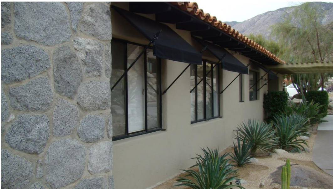
Metal Casement Windows on Front elevation
