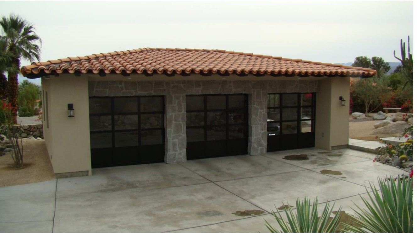
Non-Contributing Three-Bay Garage Building with Barrel Tile Hip-Roof Built in 2010. The New Garage Emulates the Main Residence in Design and Materials.
