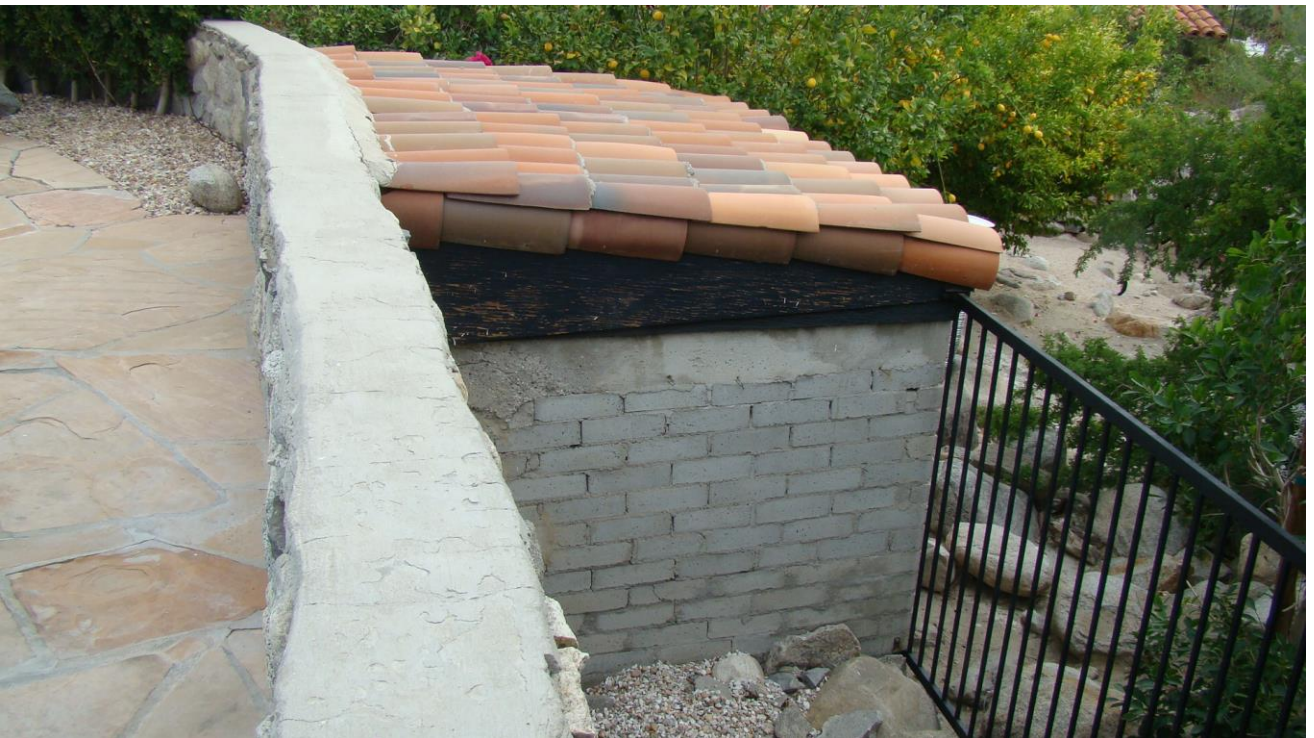
Non-Contributing Pool Equipment Building with Barrel Tile Shed Roof
