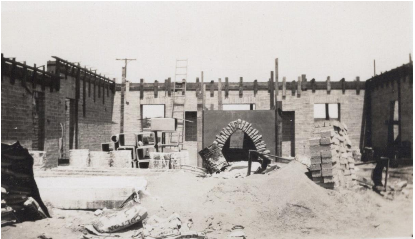
The Snyders were so proud of their new desert home they documented its construction in a series of remarkable images. This view looking north shows the rustic stone fireplace and north exterior wall beyond. (Courtesy of Mary Kummings and Steve Scott)
