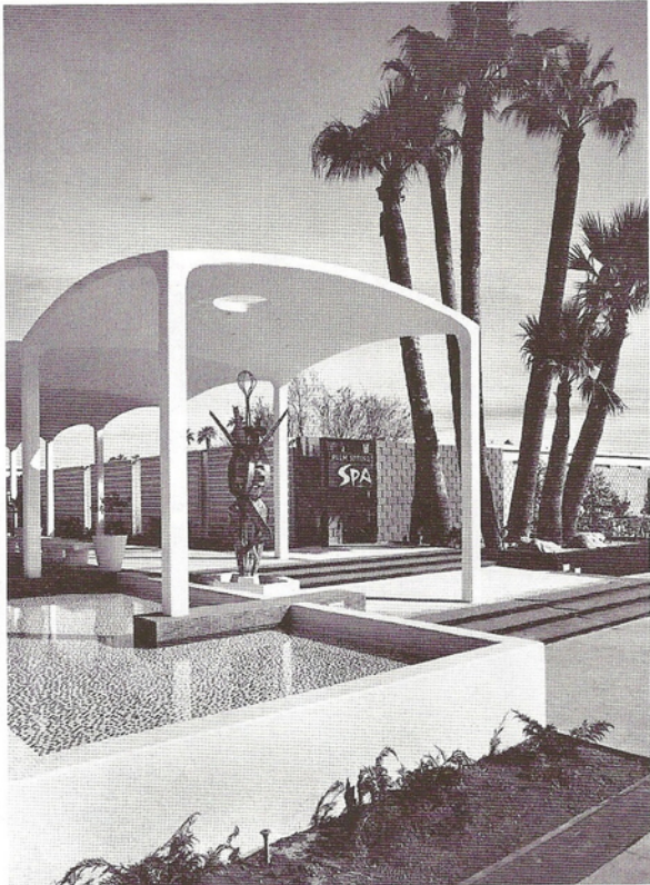
The first thin-arch, post-tension concrete colonnade to be built in California, designed by Wexler & Harrison.
