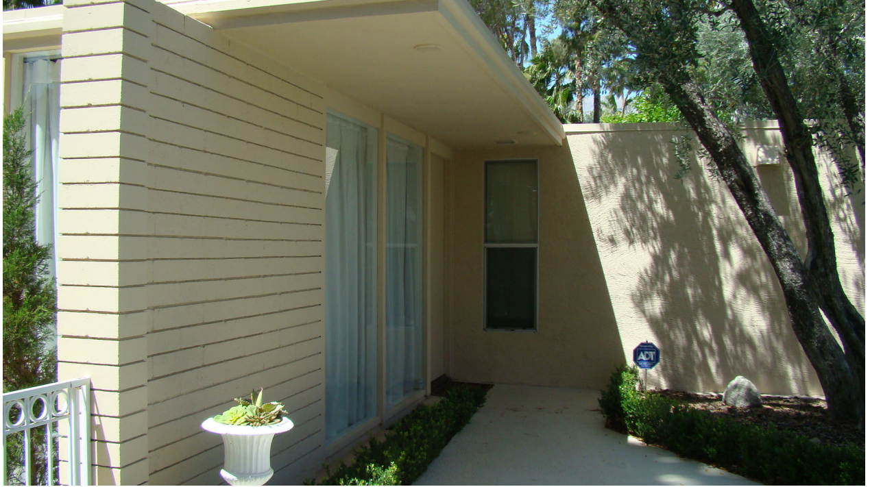
Figure 11. Roof eave detail designed for sun control
