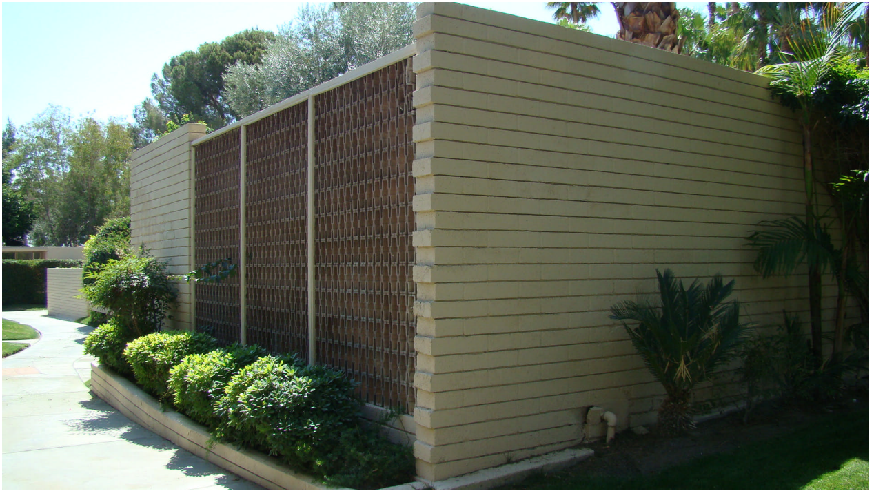
Figure 7. Concrete screen block wall and block detail
