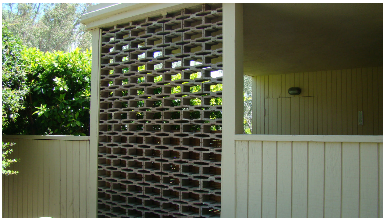
Figure 5. Occasionally, and possibly in conjunction with Bachelor units only, Cody's concrete block design is laid horizontally creating an interesting variation of the pattern.
