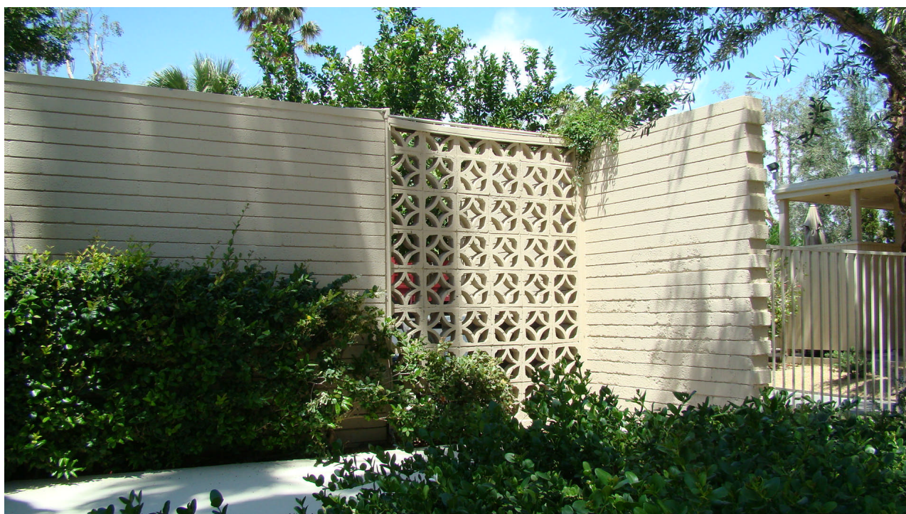
Figure 6. The RCCW condominium complex also sees use of the “Empress” pattern concrete screen block to add more privacy to the pool and cabana area. While well-executed, and appropriate for the time period, this block may have been added later.
