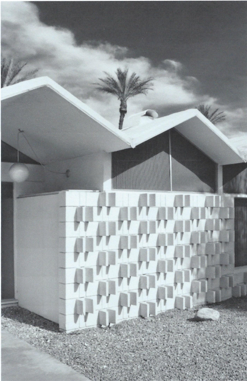
Folded plate roofs are one of the community’s distinct architectural features.
