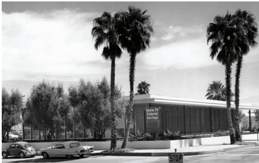
A cantilevered concrete base makes the building appear to "float."
