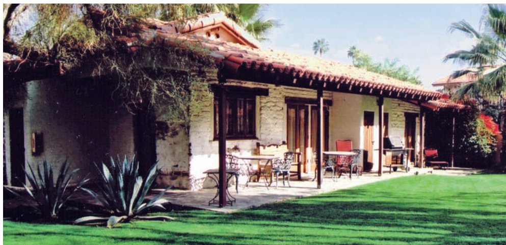
The Adobe House embodies the distinctive characteristics of the adobe method of construction, using sun-dried clay masonry units laid up in thick walls by hand in an unreinforced manner.
