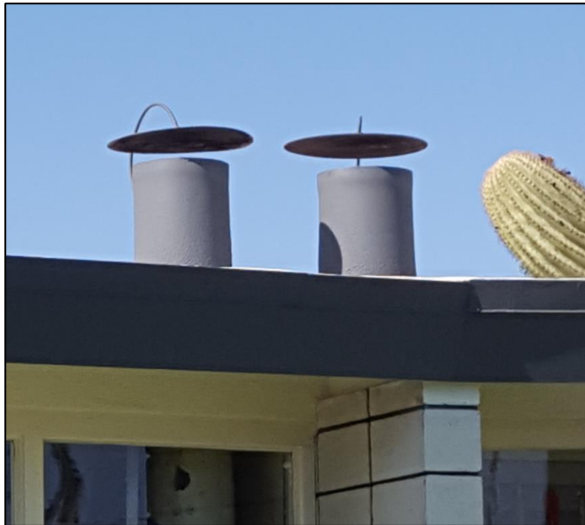
Round chimney flues are topped by unusual “pancake” spark arrestors.
