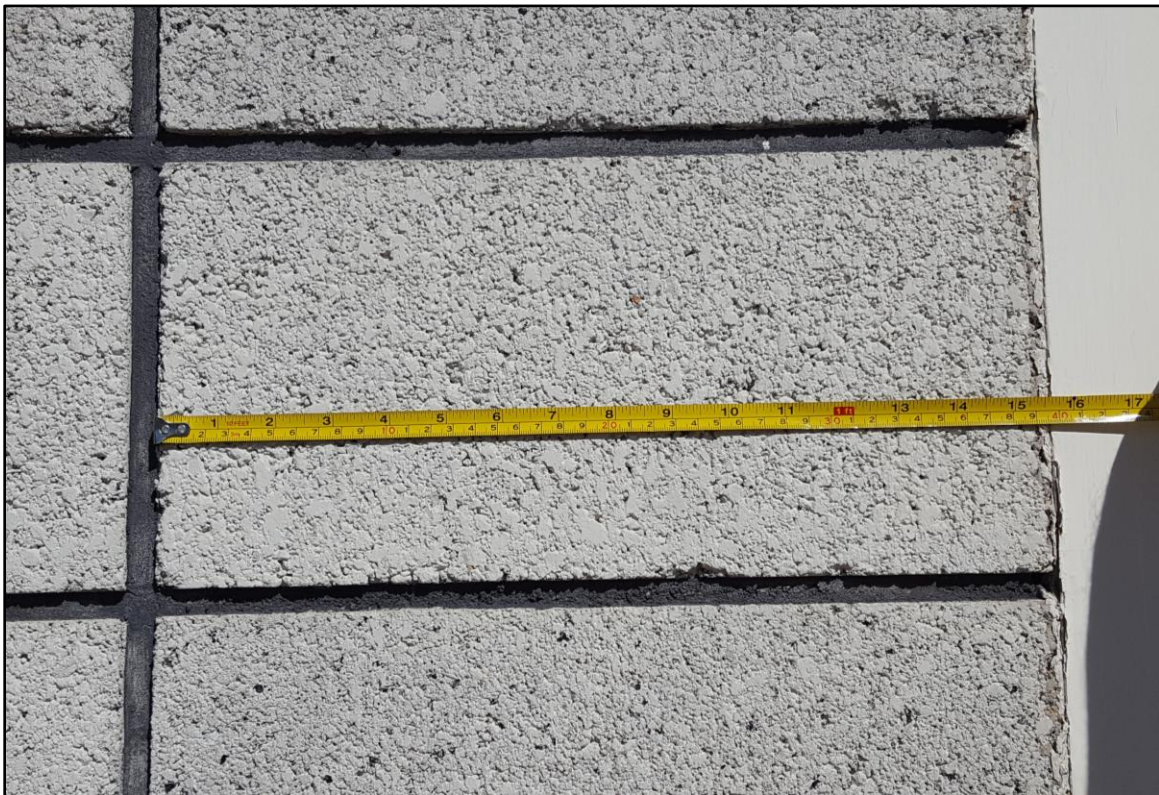
8"x8"x16" concrete block and colored mortar.
