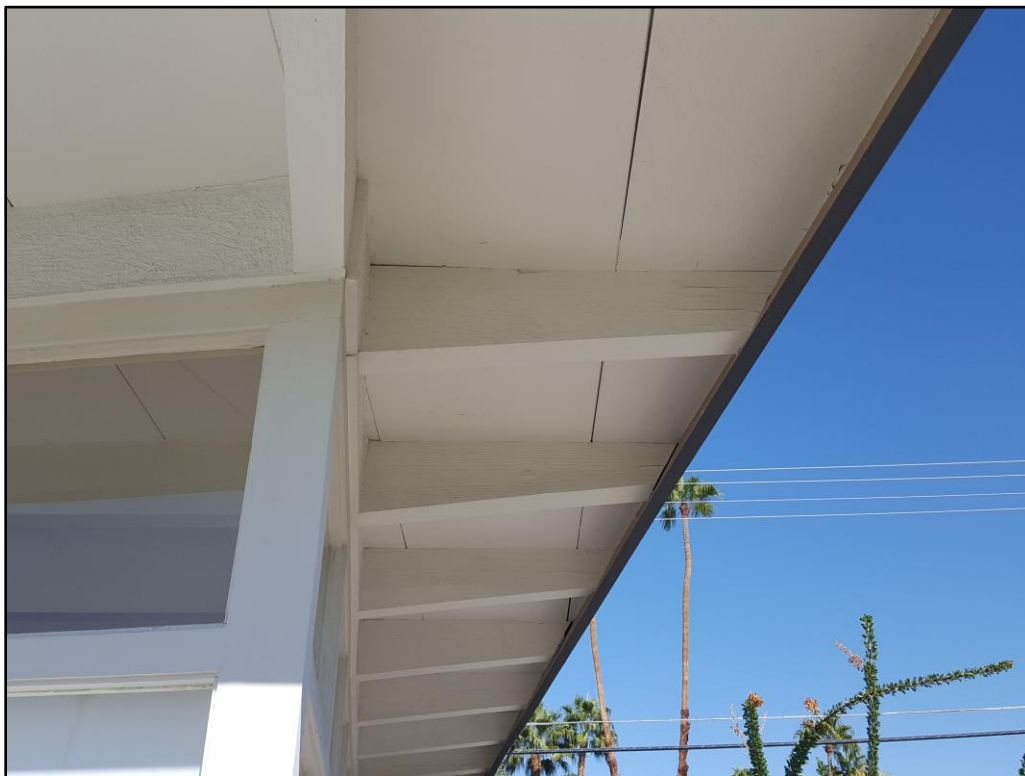
Detail of deep eave and tapering beams.
