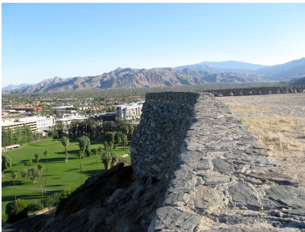
Looking south showing wall structure. (Author photo, November 2018)
