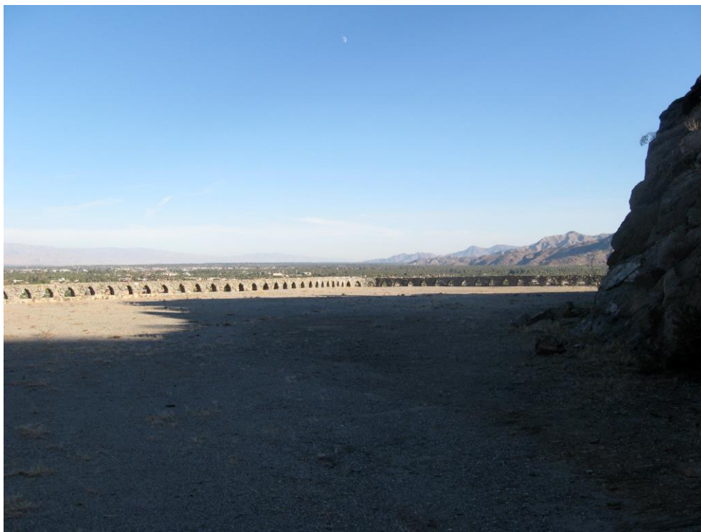
General view looking south. (Author photo, November 2018)
