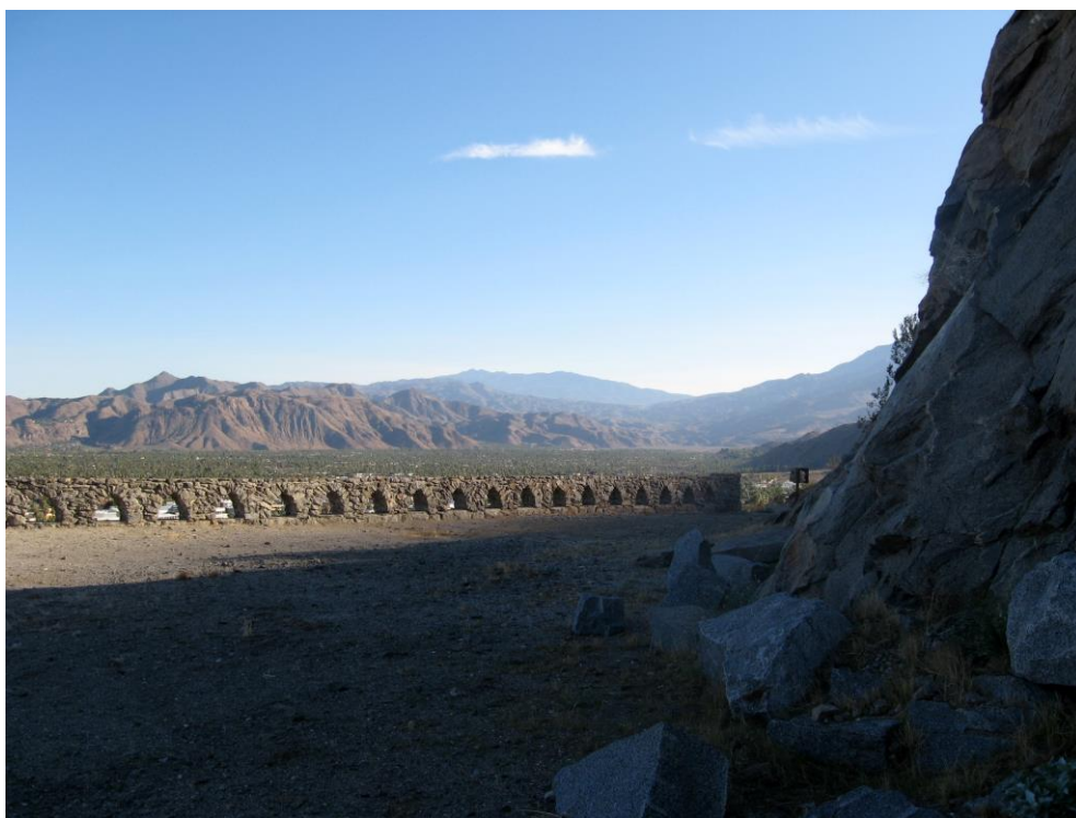
General view looking south. (Author photo, November 2018)
