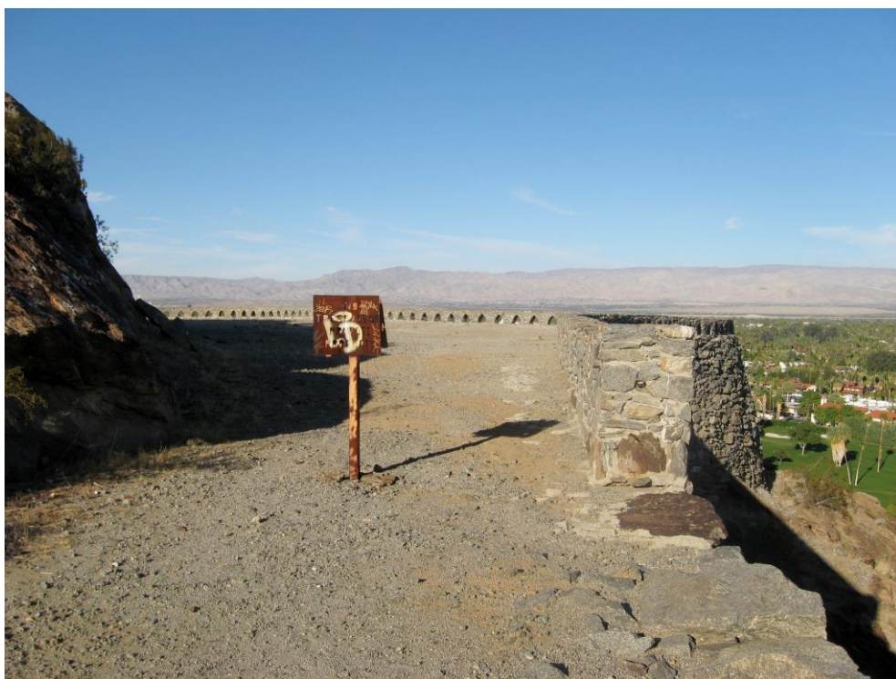
Inspiration Point southern entrance looking north. (Author photo, November 2018)
