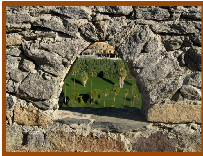
Above: Stacked stone wall detail.
