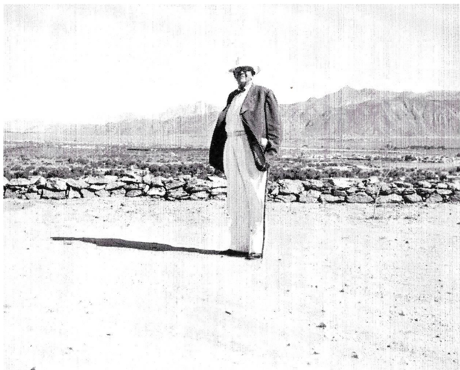
Tom O'Donnell stands on the newly-completed building pad for Ojo del Desierto. (Courtesy of Tracy Conrad)
