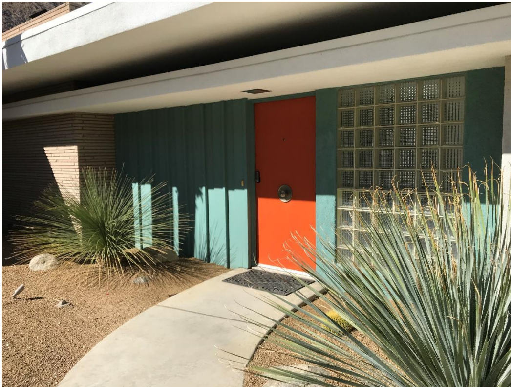
Arizona sandstone, board-and-batten, and glass block at the entrance.
