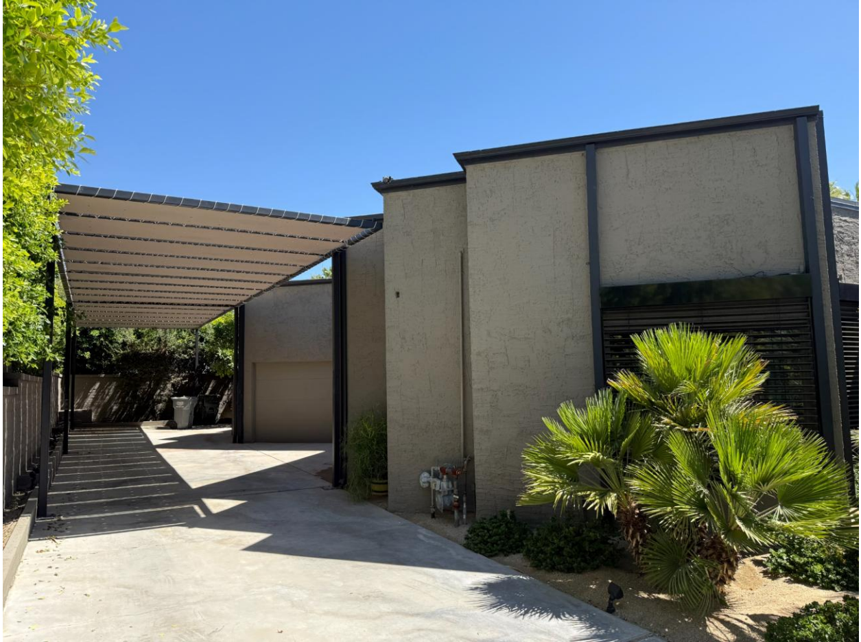
West elevation (driveway) showing the continuous parapet, canvas-covered carport, reflecting pool wall, and surviving 1946 garage wing. Photograph by author, 2026.
