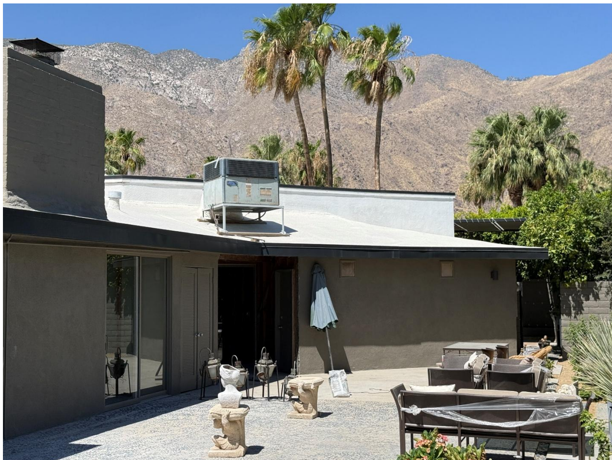
The house against the San Jacinto mountains, its flat roofs and parapet seen from the garden, with a rooftop cooling unit.
