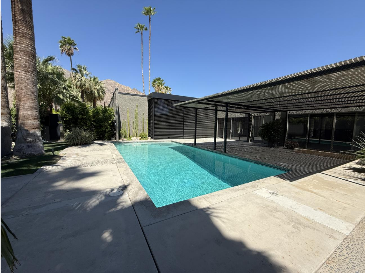
The pool and rear elevation from the opposite corner, the run of the trellis and the wall of sliding glass.
