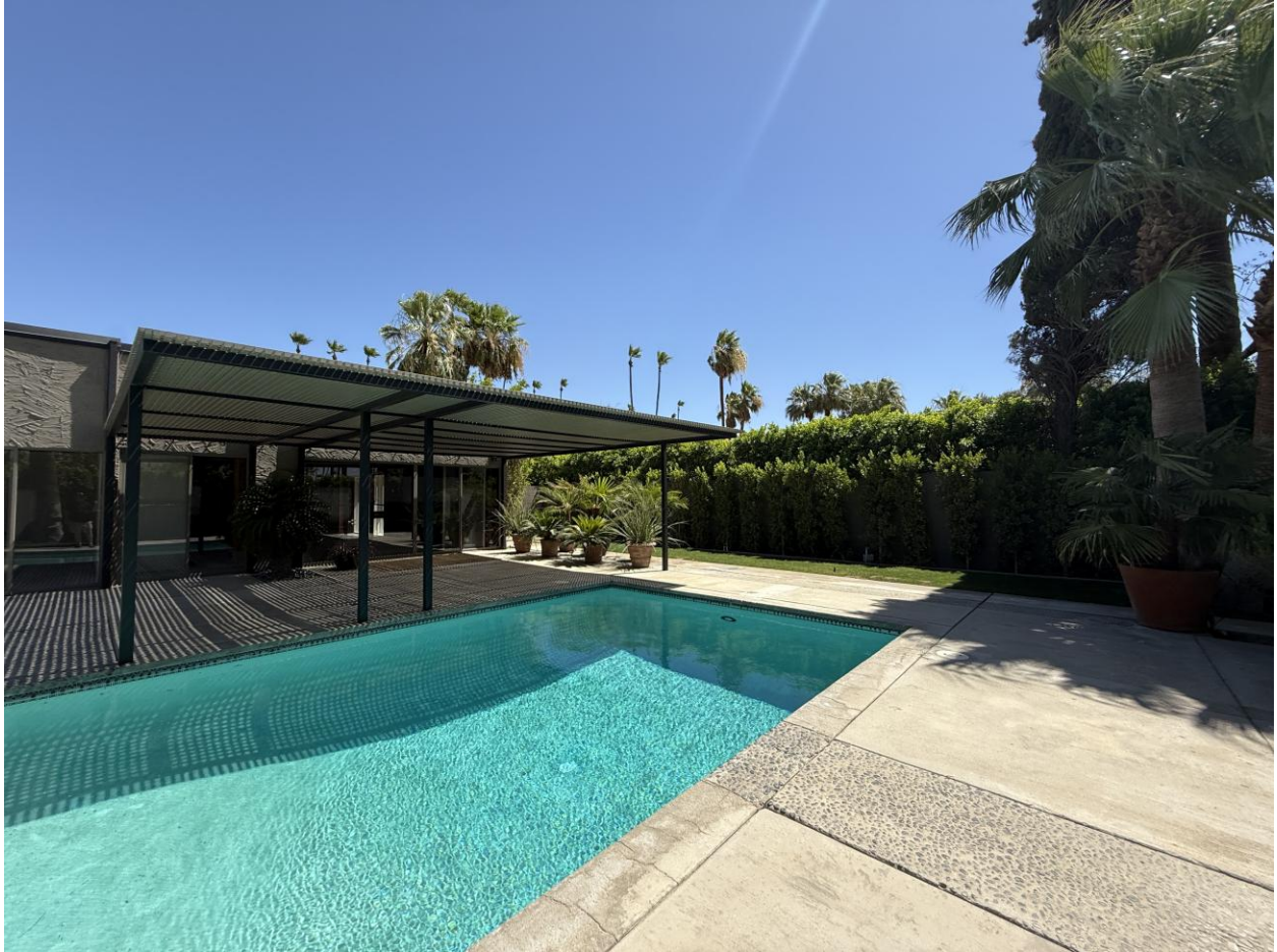
The pool and the steel-and-mesh shade trellis over the deck, the wall of sliding glass beneath it, clipped hedge and palms along the rear.
