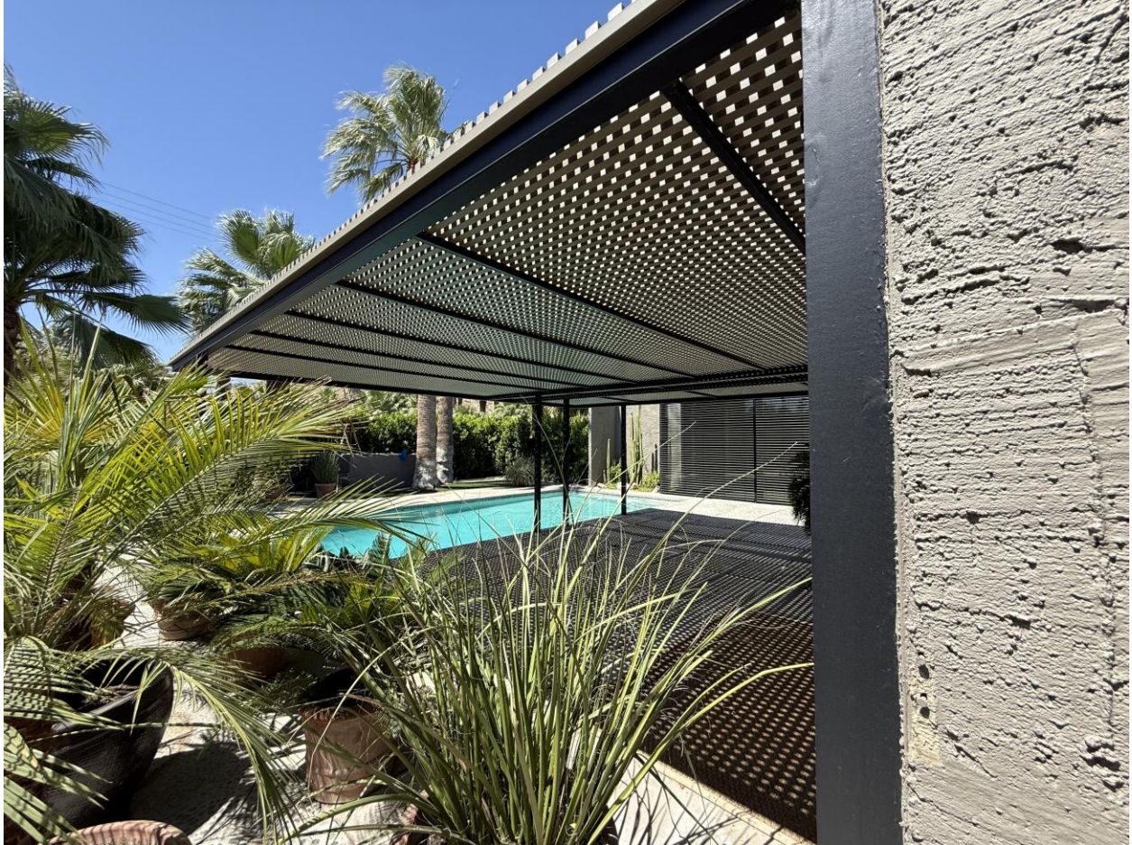
The perforated-metal shade trellis over the pool deck, the pool and garden beyond.
