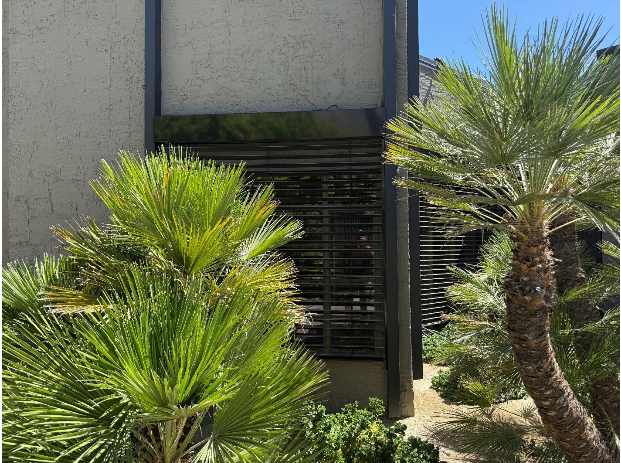
The tall west window screened in horizontal louvers, set into the driveway elevation.
