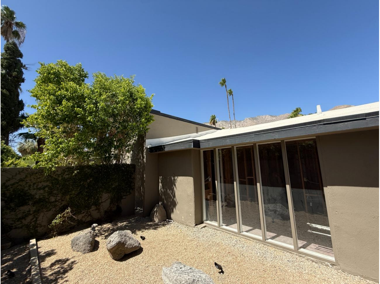
East elevation showing the 1961 bedroom addition, floor-to-ceiling fixed windows, and enclosed view court. Photograph by author, 2026.
