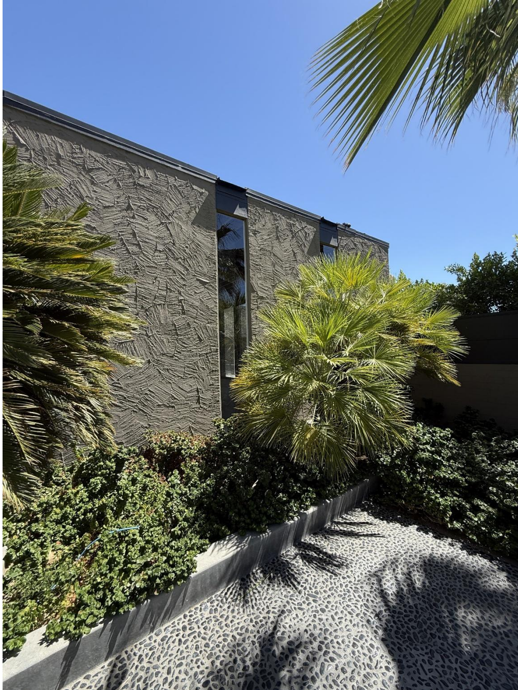
The tall street volume, its narrow windows cut as vertical slots up the sculptural troweled wall.
