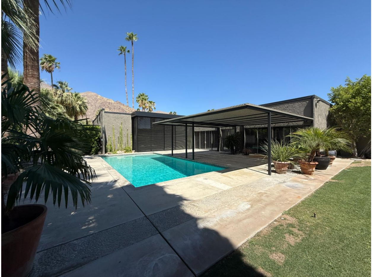
Front garden, original 1950 Paddock swimming pool, living pavilion, and steel shade structure viewed toward the residence from the southeast. Photograph by author, 2026.
