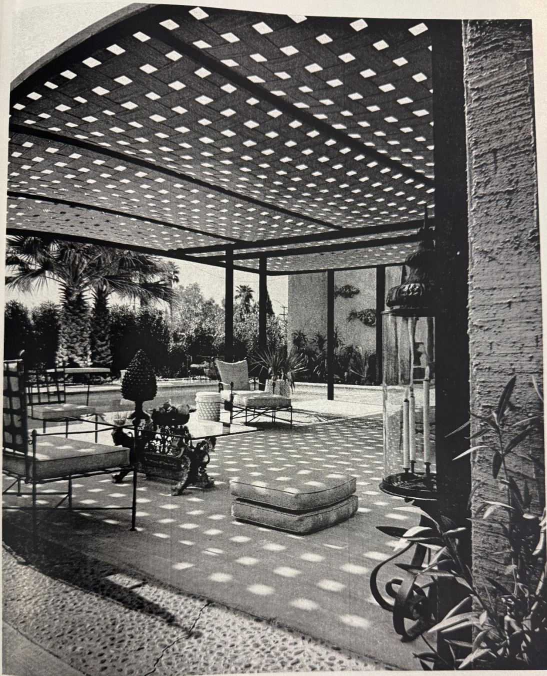
The Front Pool Terrace is covered with a canvas lattice. It is made of stitched beige canvas supported by black-brown steel columns. The furniture is from Italy and upholstered in yellow plastic. The terra cotta stools and ornaments also came from Italy. The coffee table was made from a Sicilian donkey cart.
