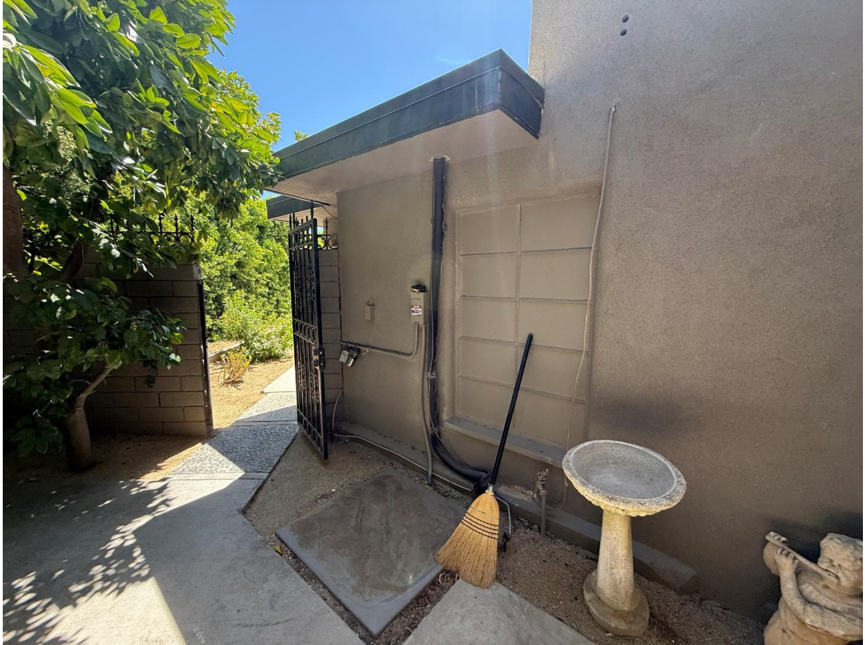
A service corner at the north side, an ornate iron gate opening to the garden, with electrical panel and hose bib on the stucco wall.
