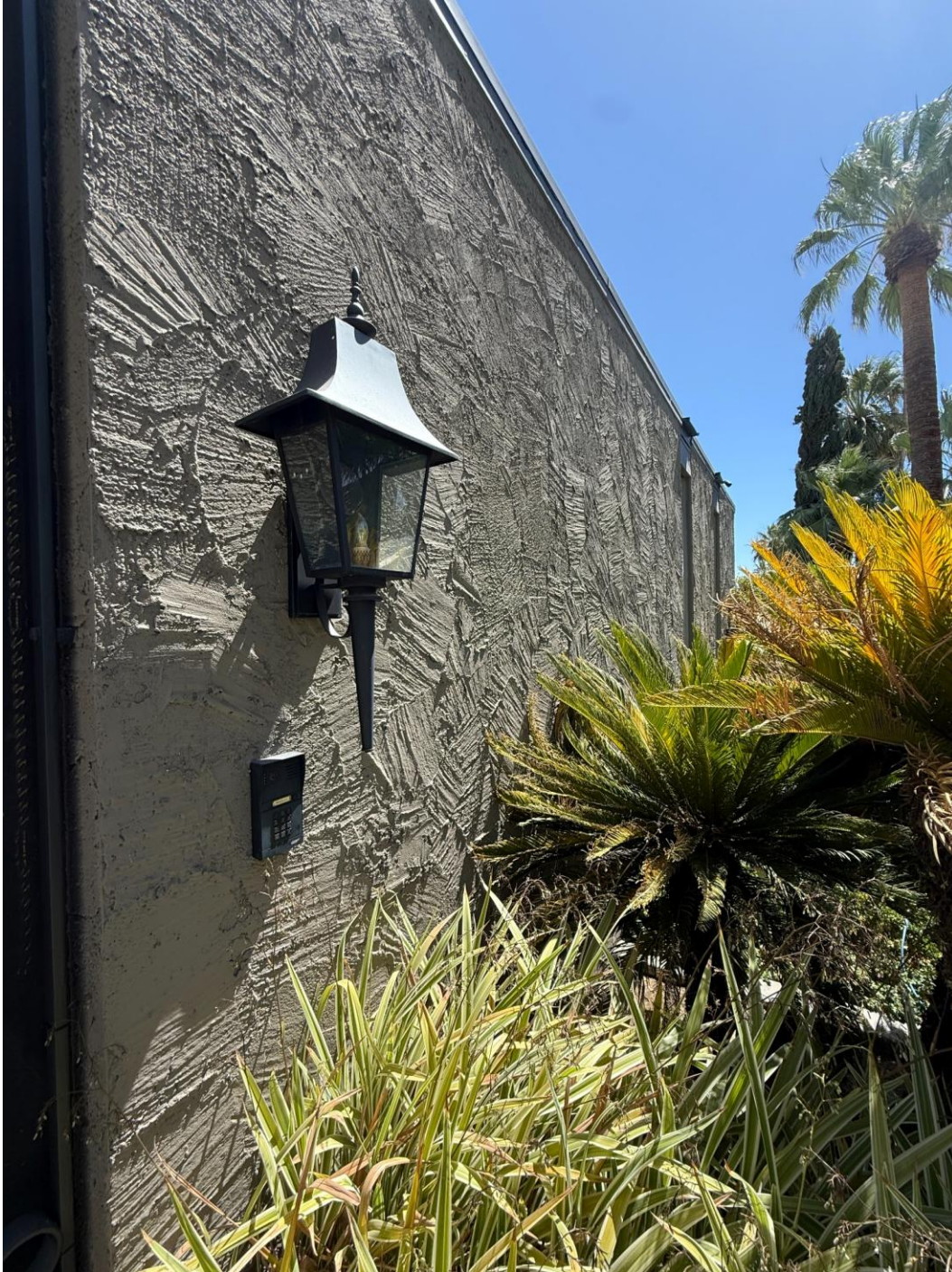
Detail of the sculptural hand-troweled cement-plaster finish on the public façade, with original iron lantern. Photograph by author, 2026.
