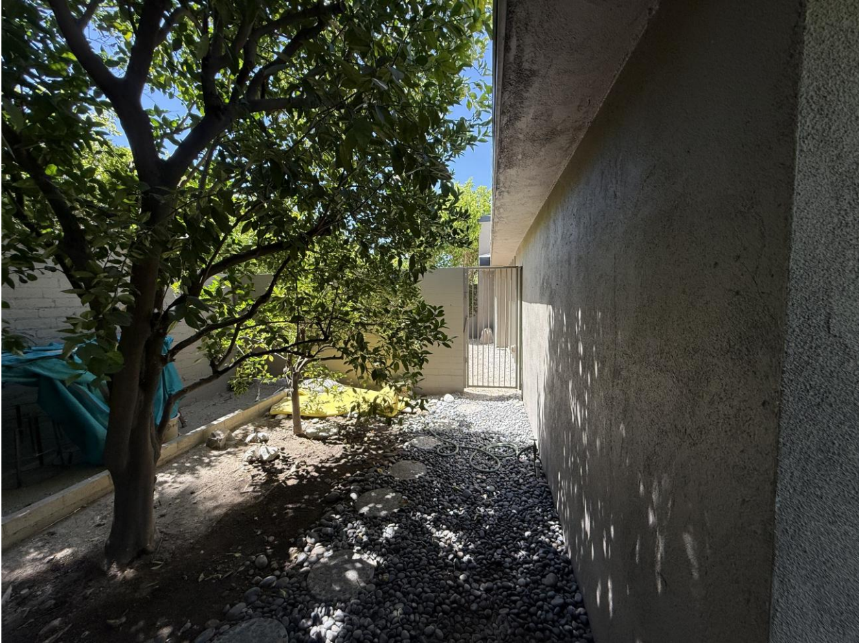
The narrow north side yard, a citrus tree over a bed of river rock, a steel pedestrian gate in the painted block wall.
