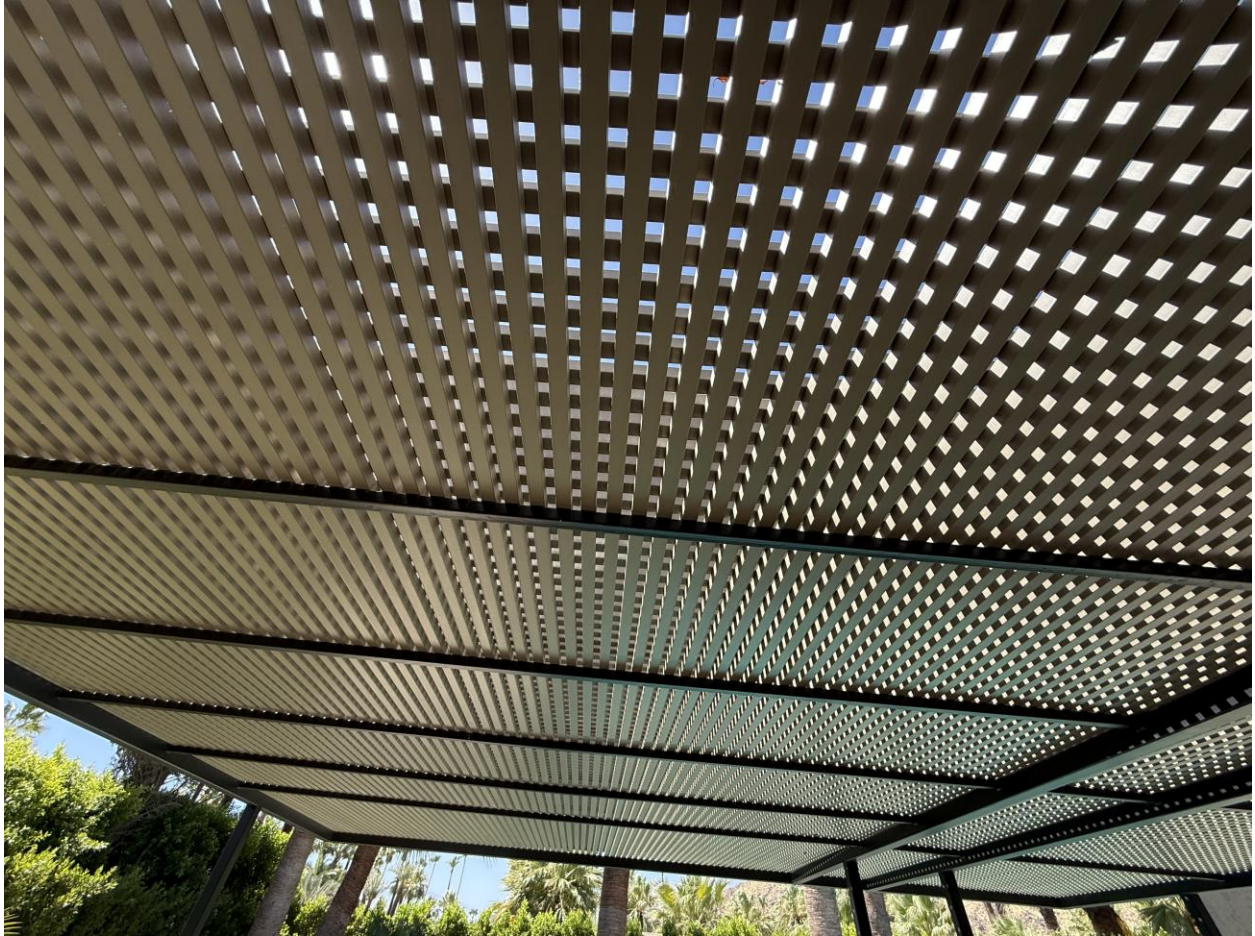
The underside of the shade trellis, its open grid laid against the sky.
