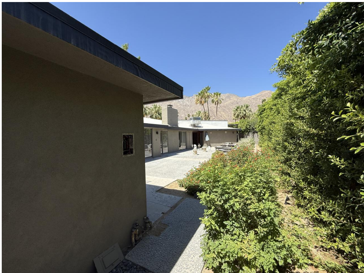
A service corner at the north side, the electrical panel set into the blank stucco wall, the pebble-aggregate walk running back toward the garden terrace and the mountains beyond.
