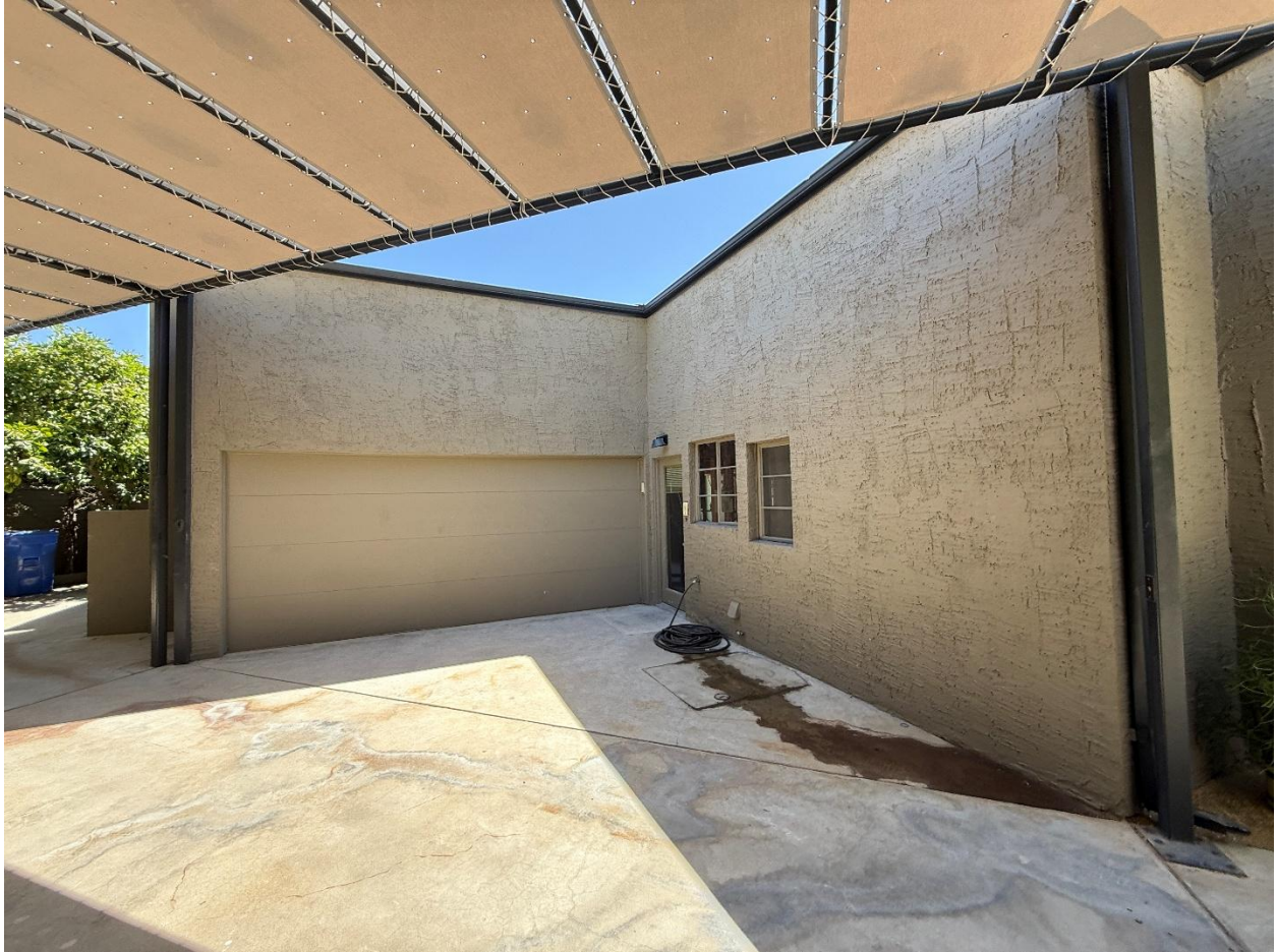
The parking court at the drive's end, the garage and 1946 service wing beneath the steel-framed shade structure.
