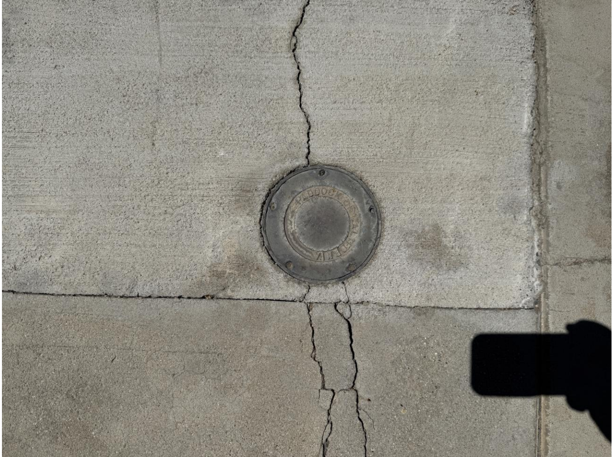
A bronze deck fitting stamped “Paddock of California,” set flush in the pool surround.
