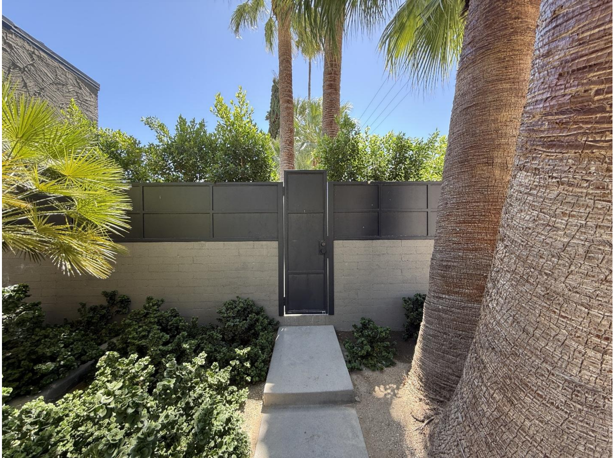
A steel pedestrian gate in a painted block wall, one of the enclosures that bring the visitor to the house by degrees.
