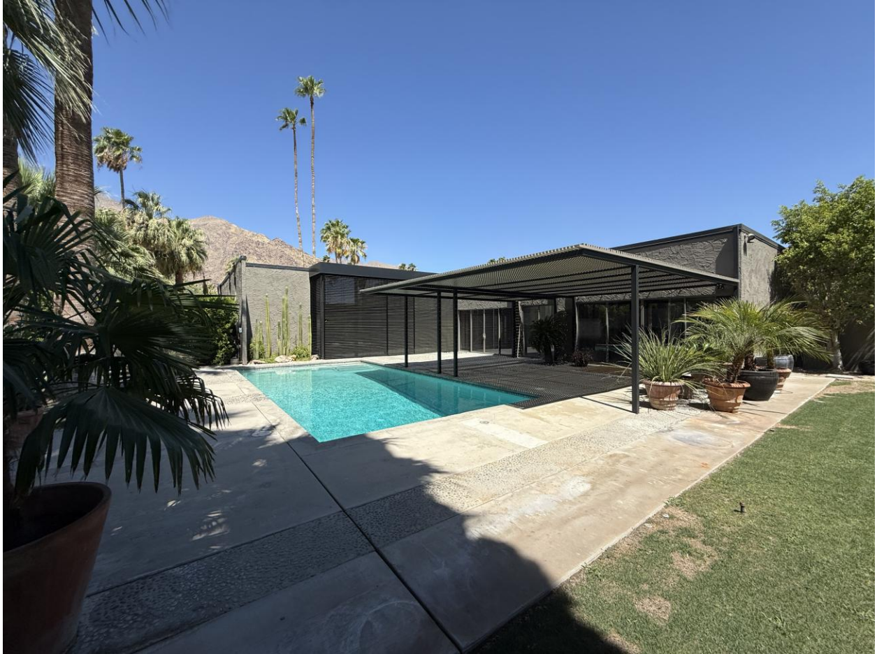
The pool and rear elevation, the louvered screen wall and the folded steel trellis over the deck.
