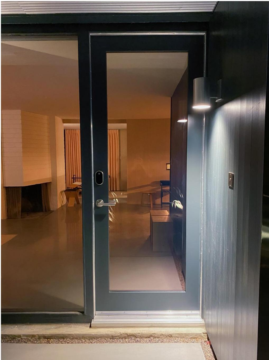
**Photo 15: October 2021 view showing newly-installed front door created to approximate the 1946 original. See photo on page 22 for comparison.
