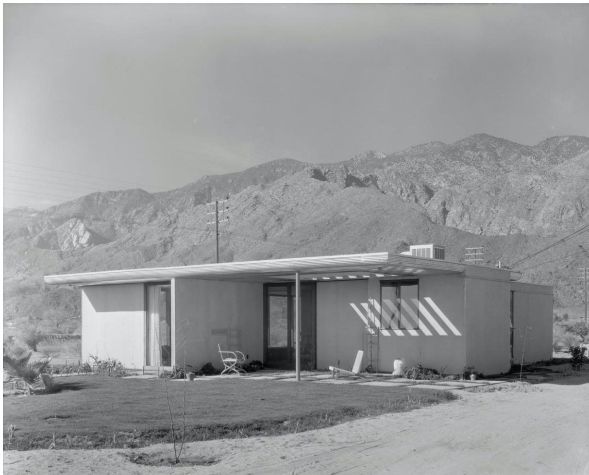
**The freshly completed Chambers Residence allows a clear view of the simplicity of its construction in Flexboard, glass and aluminum. Julius Shulman photograph.**
