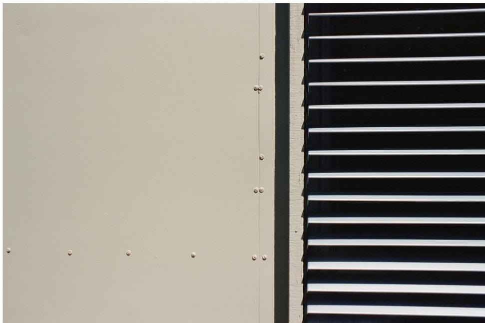
**Photo 10: West elevation detail of Flexboard attached with screws and portion of louvered bedroom window.**
