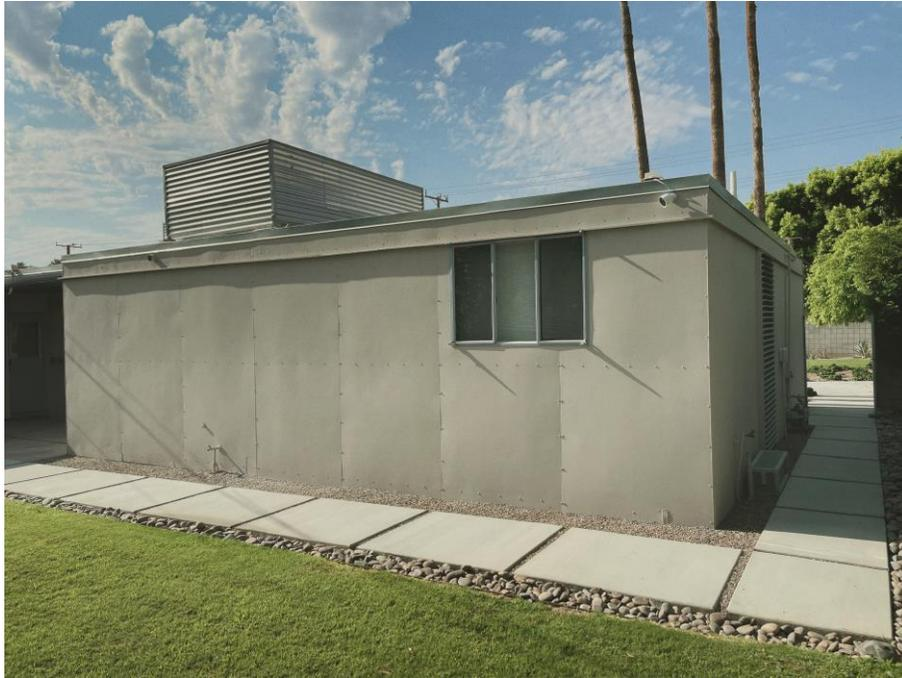
**Photo 11: North elevation showing Flexboard sheathing.**
