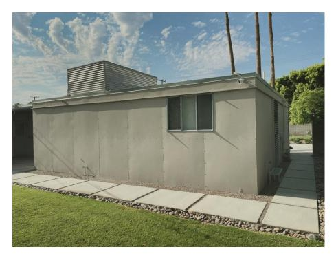
Photo 11: North elevation showing Flexboard sheathing. (Courtesy Carlos Serrao + Monica May. June 2021)
