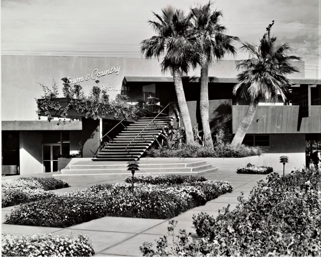
Julius Shulman photos from 1949. The fronts of balconies and overhead fascia are darker than the main stucco body of the building:
