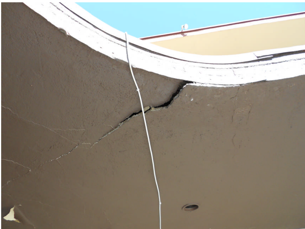
Photos 19 and 20: Severely cracked stucco under eaves in courtyard – Violations of subparagraphs A.3.ii and A.3.iv
