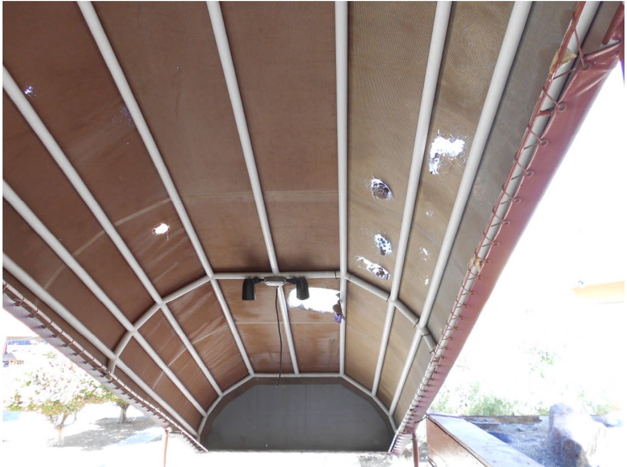
Photo 9: Deteriorating awning covering – Violations of subparagraph A.3.ii and A.3.iv.
