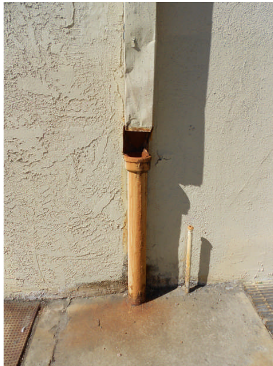
Photos 21 and 22: Severely rusted air-conditioning unit on North Indian Canyon Drive. Rusting downspouts are another systemic problem – Violations of subparagraphs A.3.ii and A.3.iv
