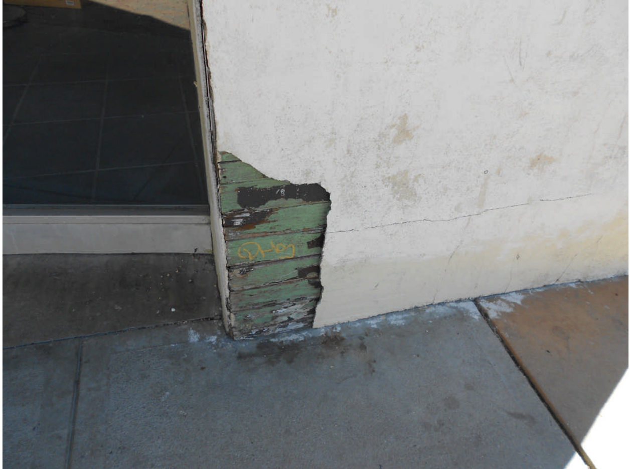
Photo 18: Missing stucco (a systemic problem throughout the complex) on North Palm Canyon Drive – Violation of subparagraphs A.3.ii and A.3.iv
