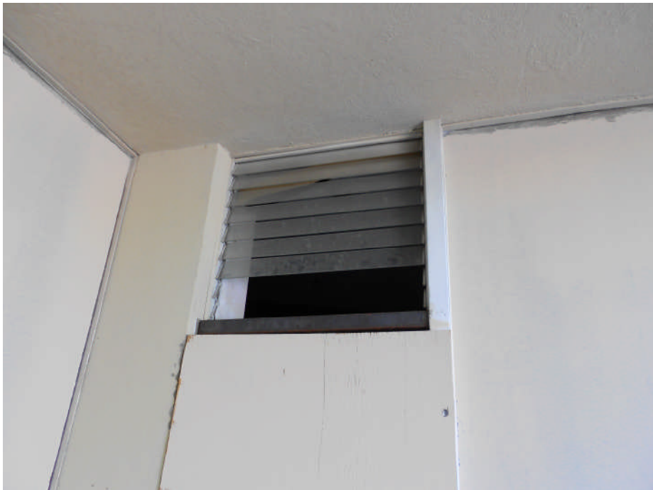
Photos 10 and 11: Broken windows and missing panes of jalousie window – Violations of subparagraph A.3.vii
