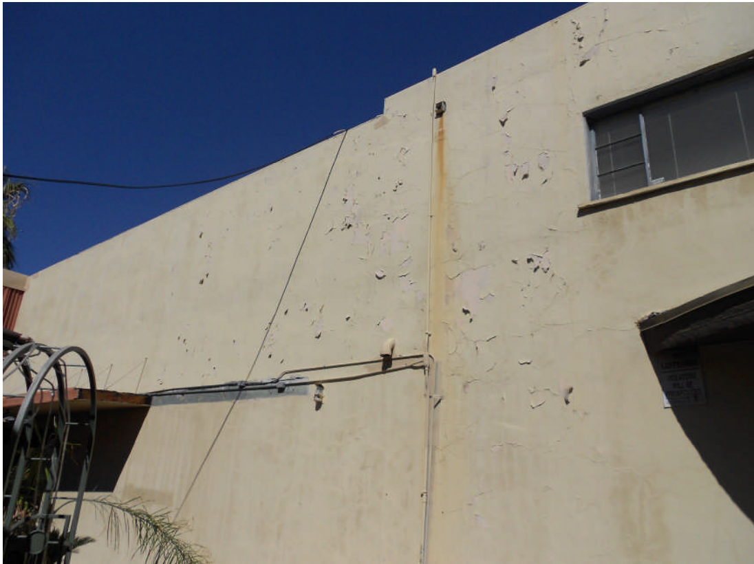
Photos 5 and 6: Peeling paint (this is a systemic problem throughout the complex) – Violations of subparagraph A.3.ii
