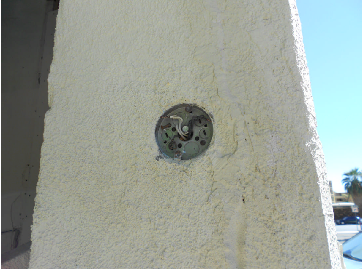
Photo 12: Uncovered electrical junction in courtyard. Although probably not electrified, “mystery wiring” is a systemic problem throughout the complex and constitutes a potential safety violation – Violation of subparagraph A.3.iv
