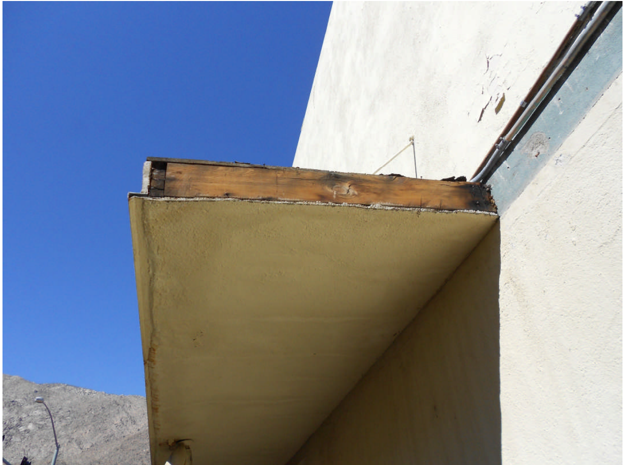
Photo 17: Missing fascia – Violation of subparagraphs A.3.ii and A.3.iv
