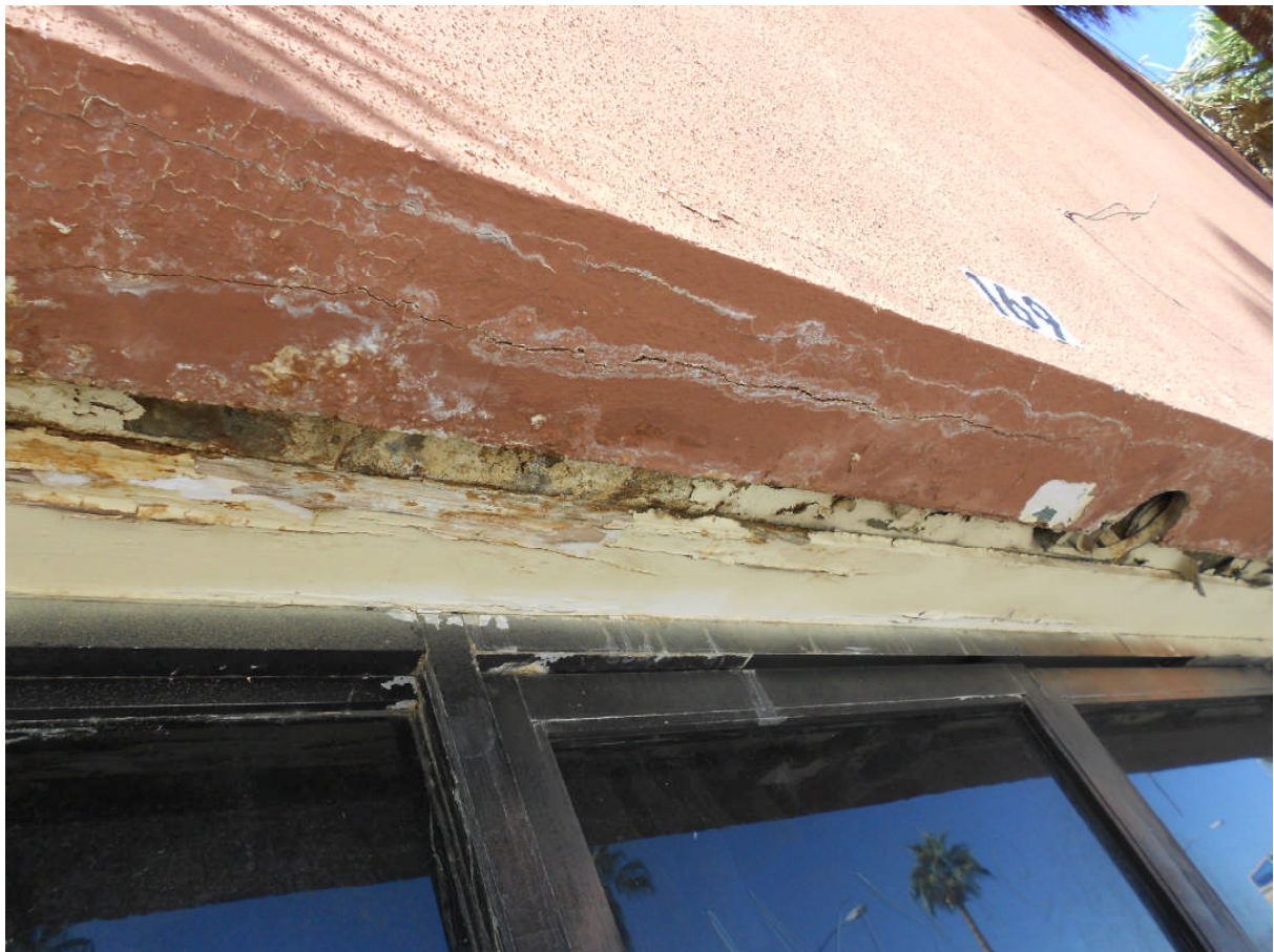
Photo 1: General deterioration of the structure (water damage) on North Indian Canyon Drive – Violations of subparagraphs A.3.ii and A.3.iv.
