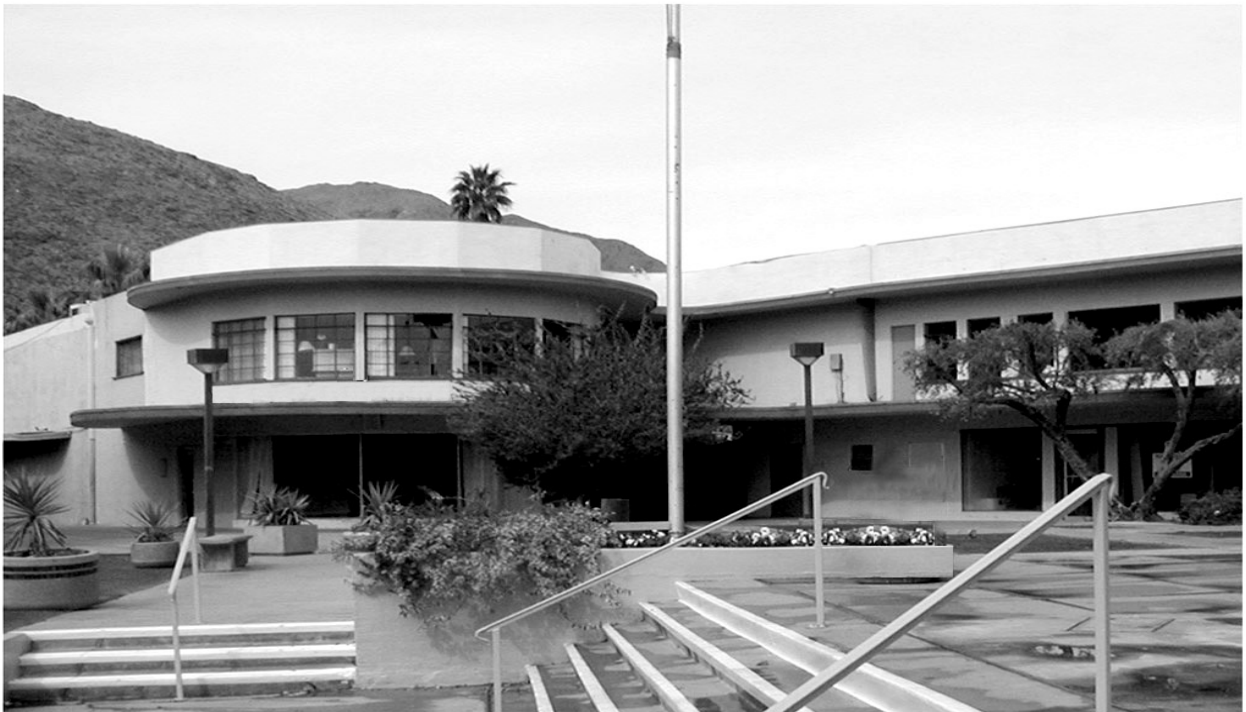
Figure 4 In this February 2000 photograph the T&CC appears to be occupied and well maintained; the landscape is manicured and paved areas are freshly washed. Under the present ownership it has been allowed to deteriorate.
