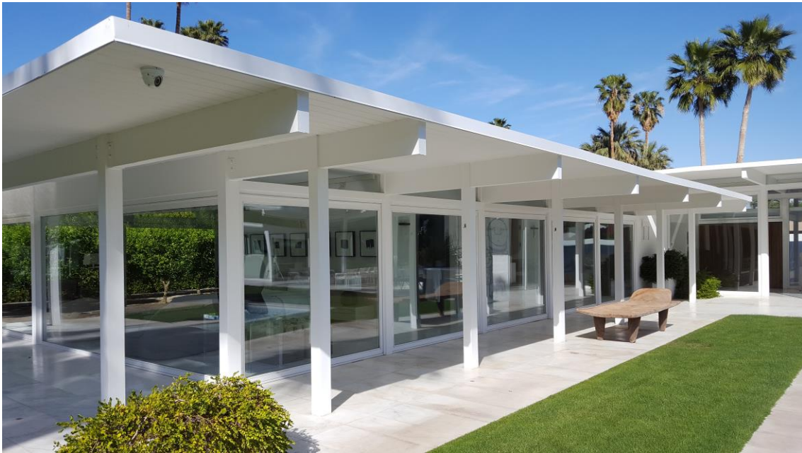
Post-and-beam construction.
