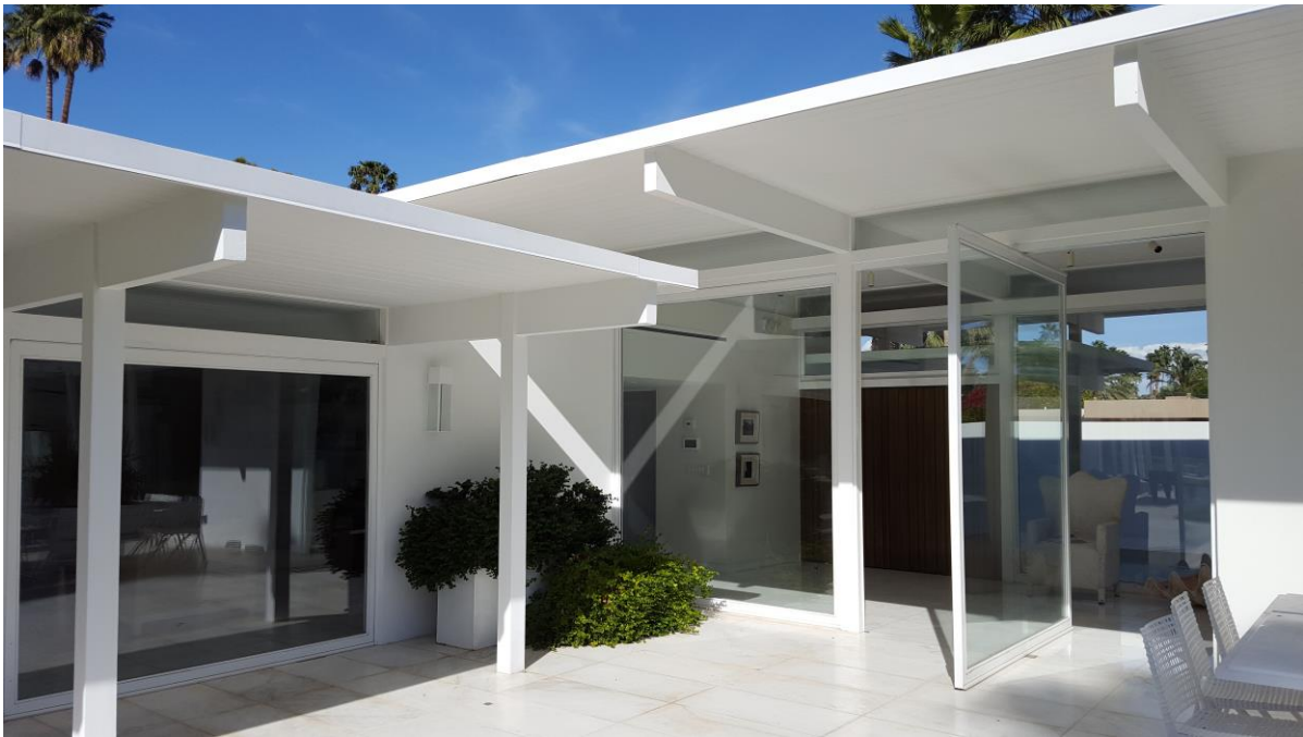
The multi-level flat roof provides visual interest and helps demarcate common areas from private areas by creating different ceiling heights. Also shown are clerestory windows and the post-and-beam construction.
