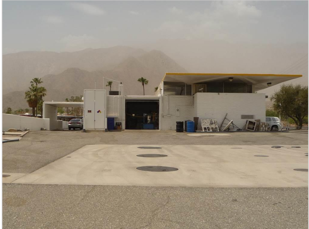
East elevation, view southwest.
