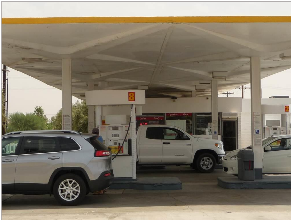
West elevation, detail of canopy, view northeast.
