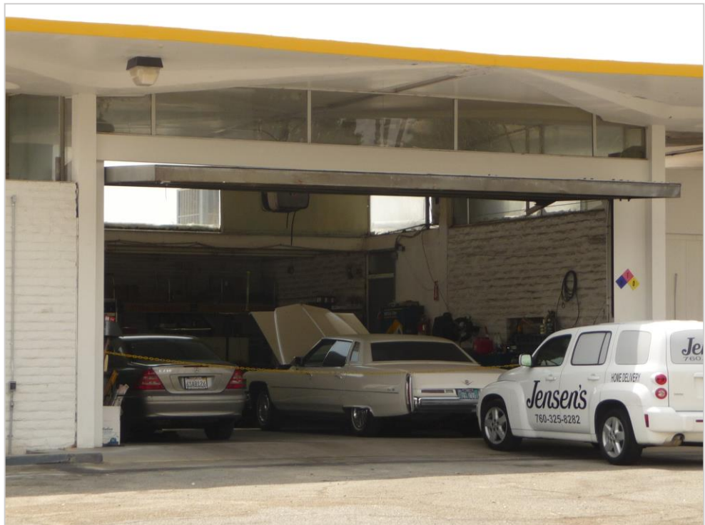
Detail of service garage interior, showing slump stone construction and clerestory windows, north elevation, view south.
