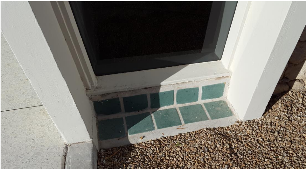
Vintage 4"x4" glazed turquoise tiles at the base of the wall on the east side of the residence.
