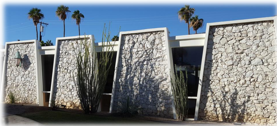
Cofferred stone piers
