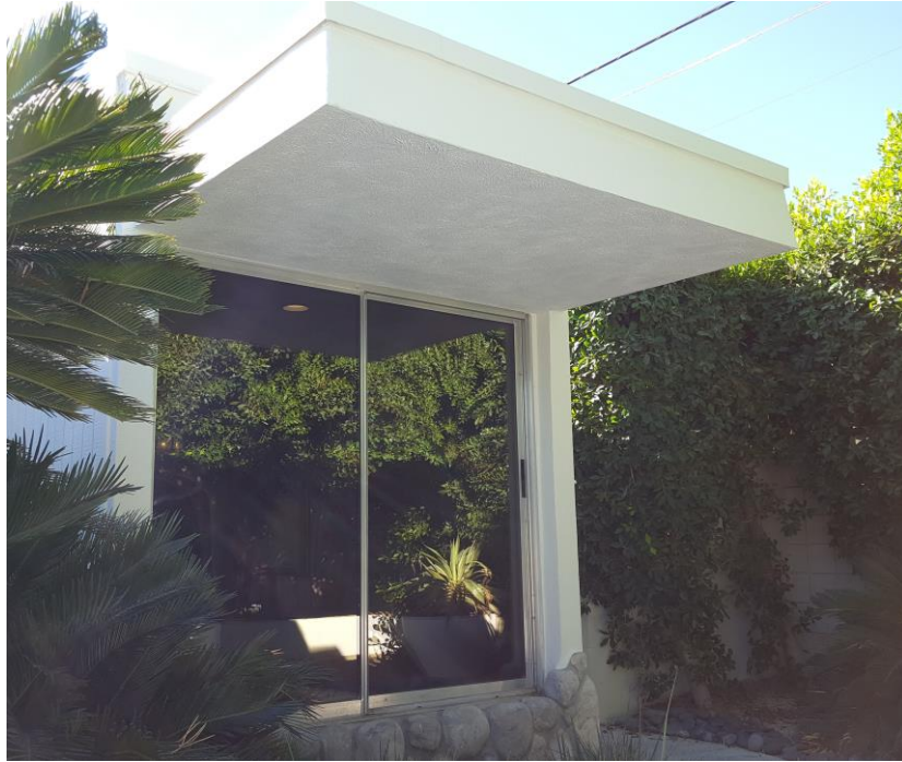
Throughout the residence's design, deep and projecting eaves moderate the solar heat
