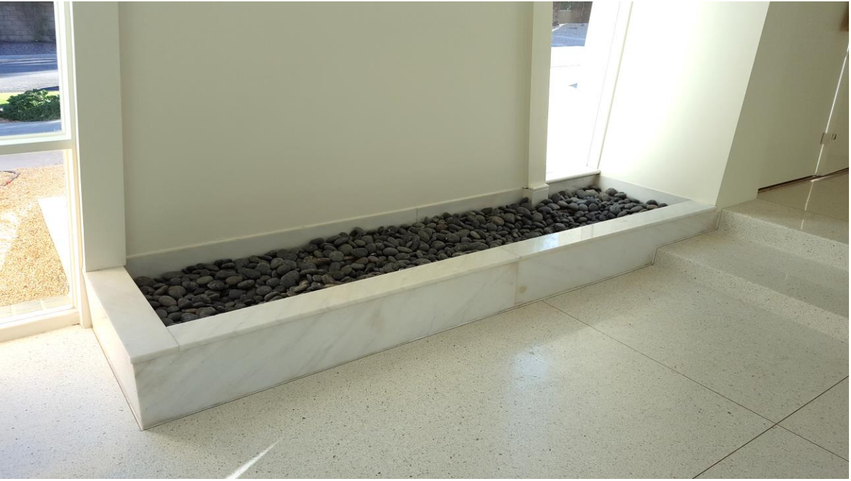
Marble-faced interior concrete planter.
