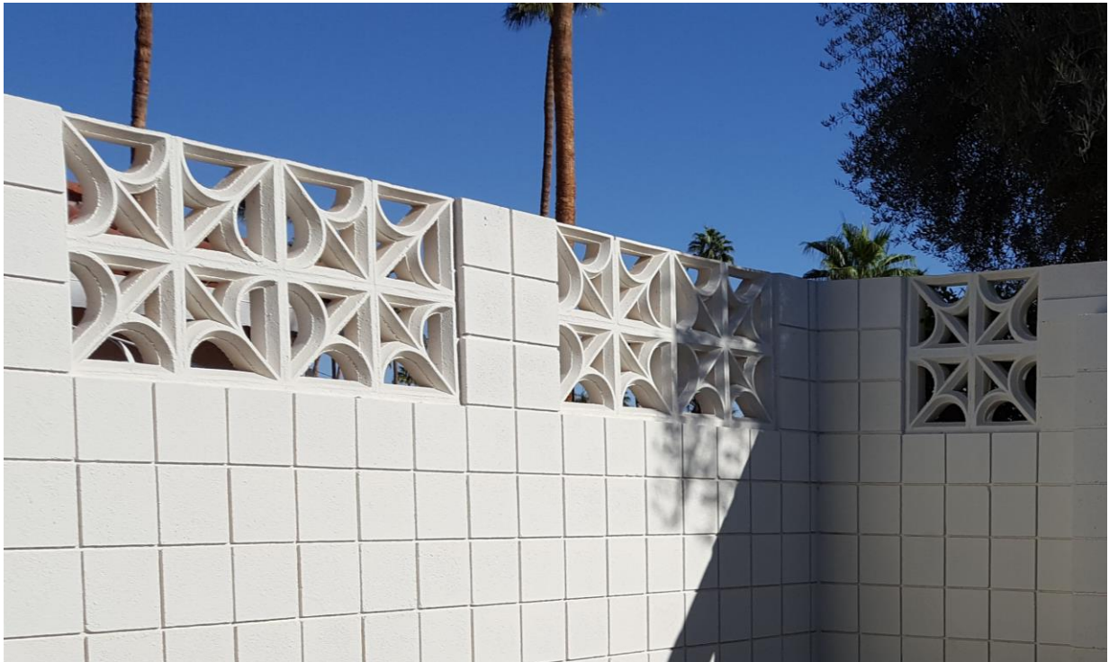
Concrete screen block in the "Sprite" pattern and 8"x8" square solid concrete block.
