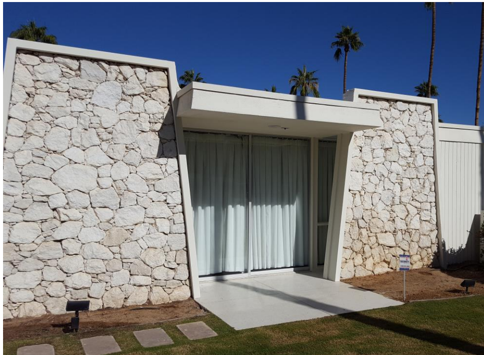
Terrazzo walkway leading to sliding glass doors on south side of residence.
