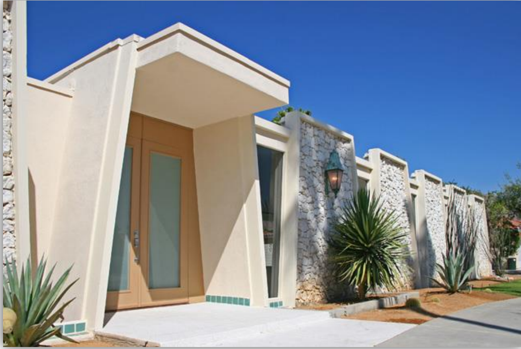
A circa 2005 photograph showing the “unsympathetic” framed glass doors which replaced the original doors. These doors were later replaced in October 2016.
