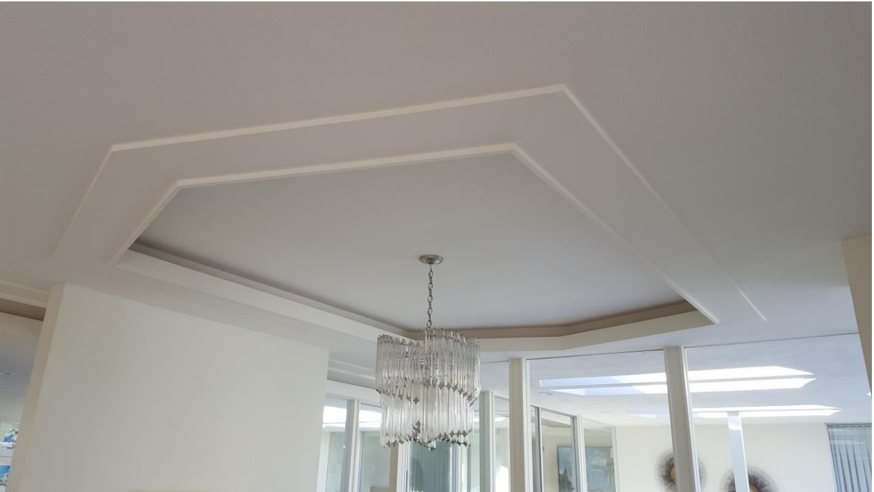
Tray ceiling over dining area. Tray ceilings can also be found in the main hallway.
