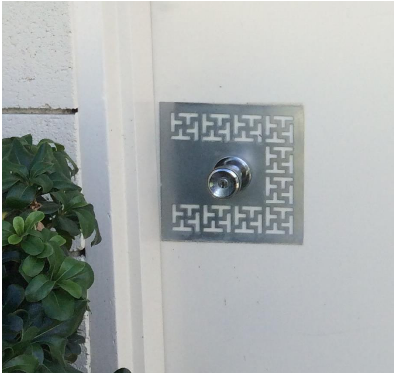
Detail of one of two types of original escutcheons (decorative plates) around door handles
