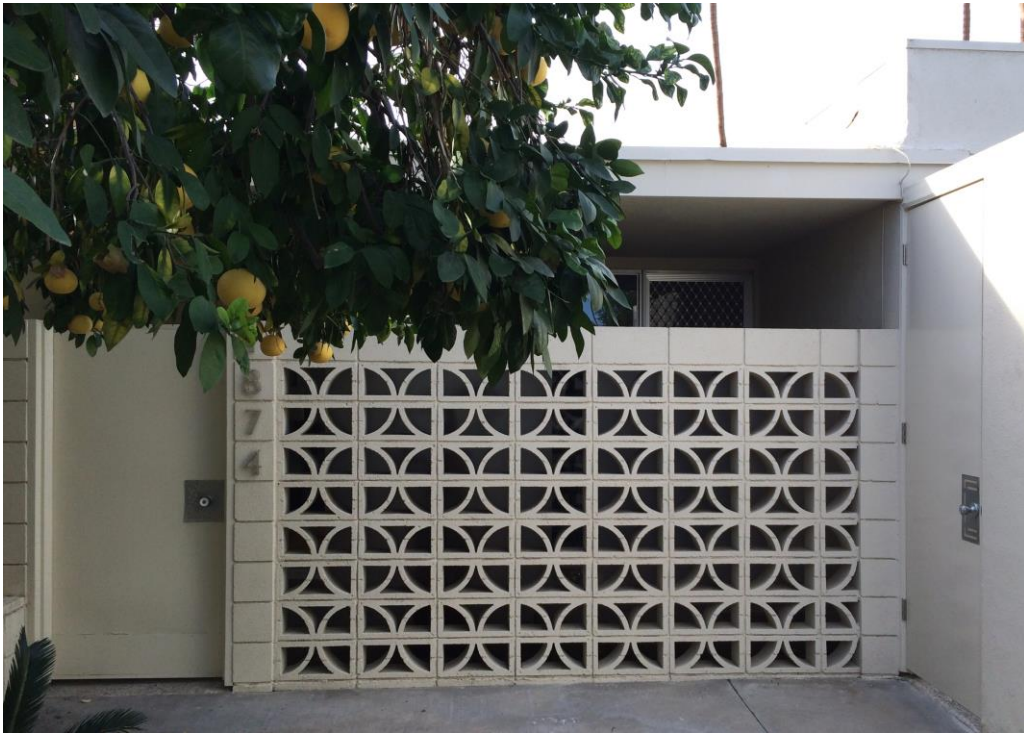
Sandcliff unit at 1874 Barona Road rear main entry showing “Four Circle” concrete screen block wall
