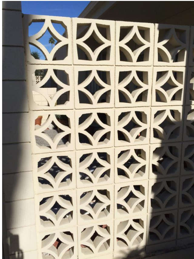
“Empress” pattern concrete screen bock
