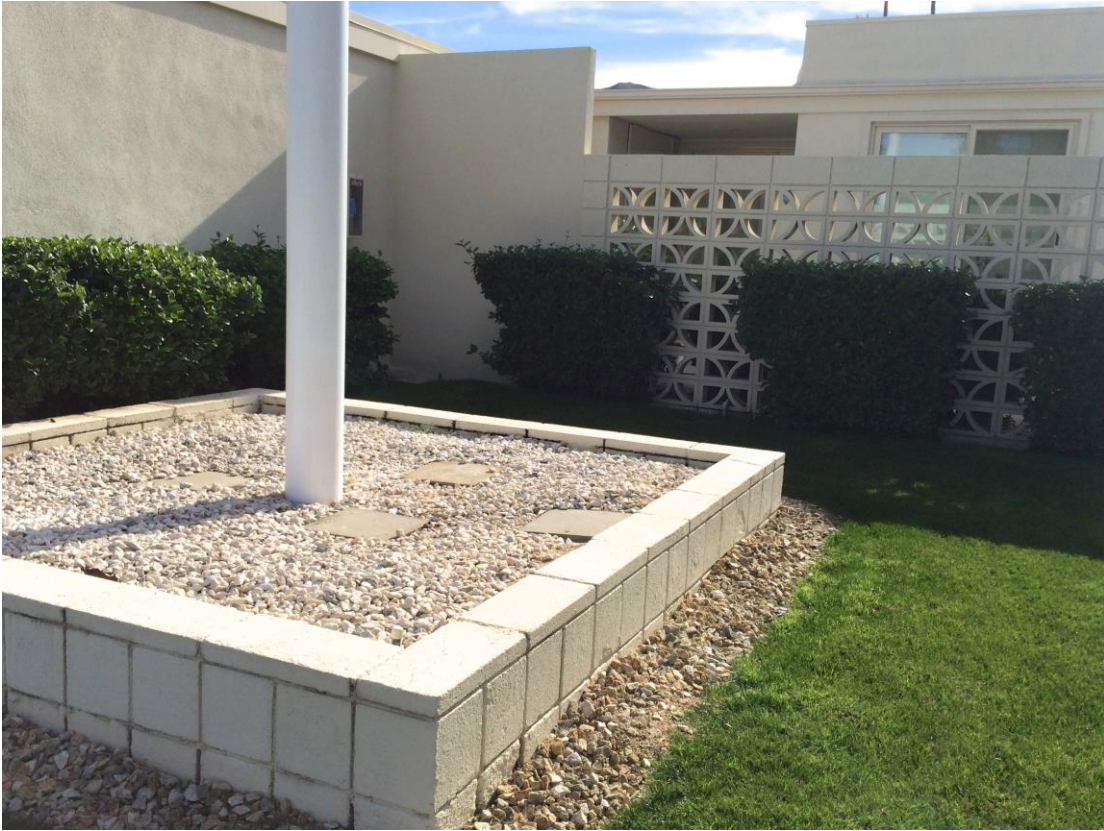
Original planter (note 8"x8" concrete block) with screen block wall in background
