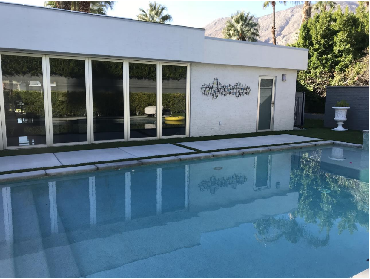
Original aluminum sliding glass doors were replaced with accordion-fold aluminum and glass doors.
