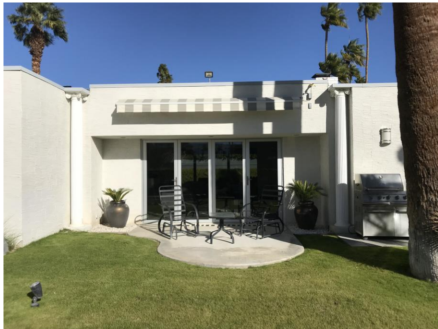
More accordion-fold doors facing Camino Norte.
