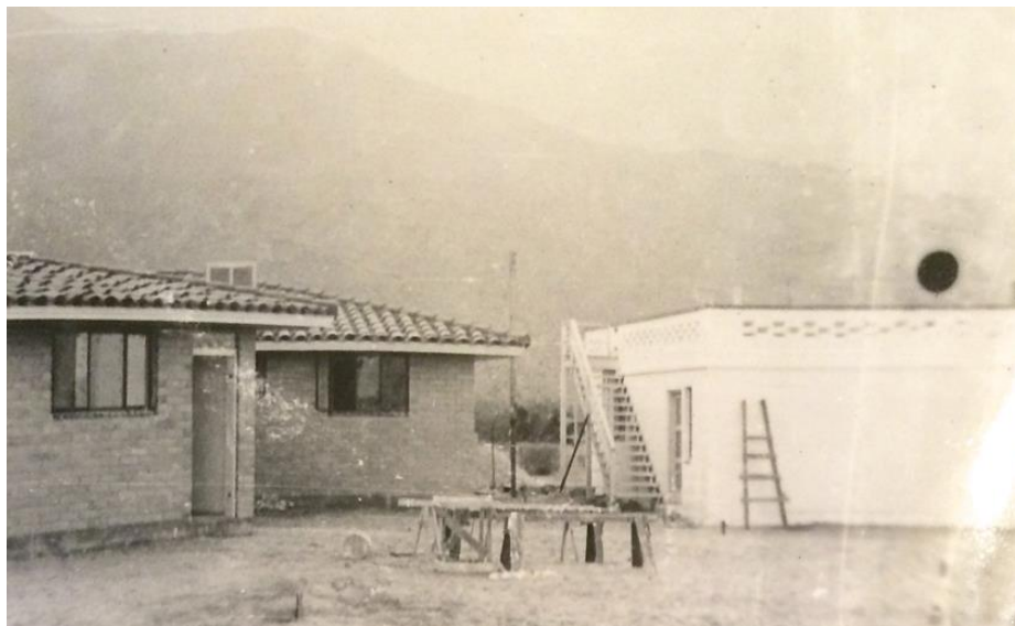
Photograph of Building 1a (right) under construction. Mildred Paul's notes read, "Evelyn completed her garage first to store all building accessories." (Courtesy Valorie Hodgert)
