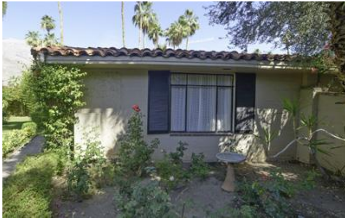
Building 1, Room 103, original window.
