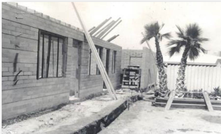
Building 4 under construction, with Building 1a (garage) to the left. (Courtesy Valerie Hodgert)
