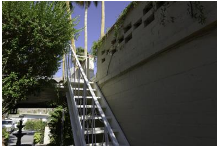
Building 1a showing the original stairs to the roof deck of garage (now office).
