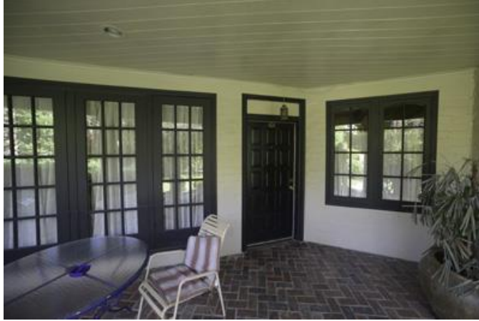
Building 1, Room 101, entry and deep porch. The door and windows have been replaced.
