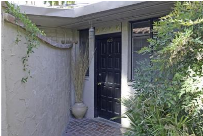
Building 1, Room 105, entry door (replaced), glass block detail and original windows.
