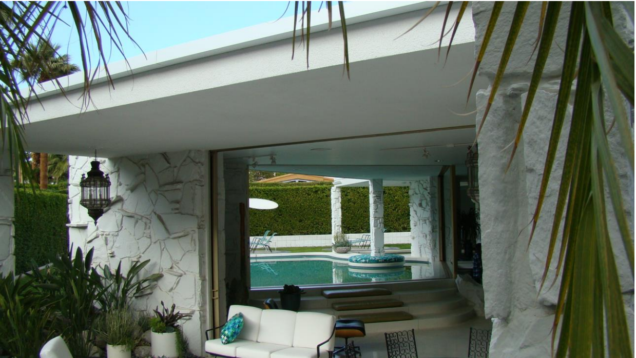
View from the patio, through the south sliding glass pocket doors and sunken living room to the pool and beyond. Also seen are the deep eaves which provide passive solar control and the effect of “transparency” when the large glass pocket doors are stowed.
