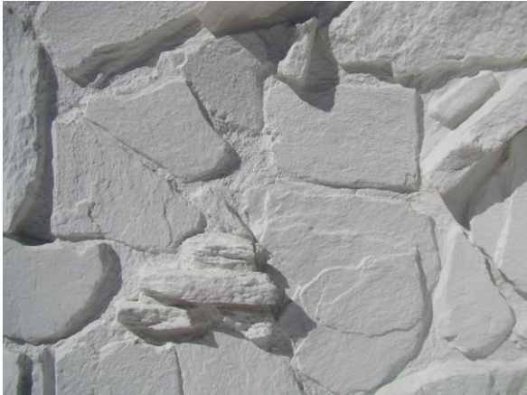
Painted stonework (historical photographs indicate stonework was painted prior to 1970)
