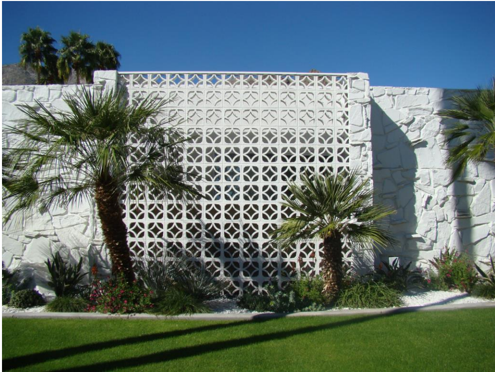
Concrete screen block wall covering windows on east façade. The “Empress” screen block pattern is discussed in detail in Appendix VIII.
