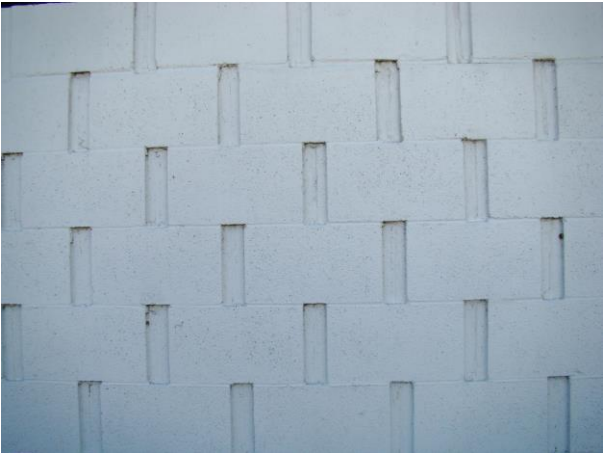
Concrete block (trade name "Shadowal")
