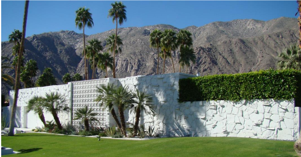
The Morse Residence’s street-side (east) façade
