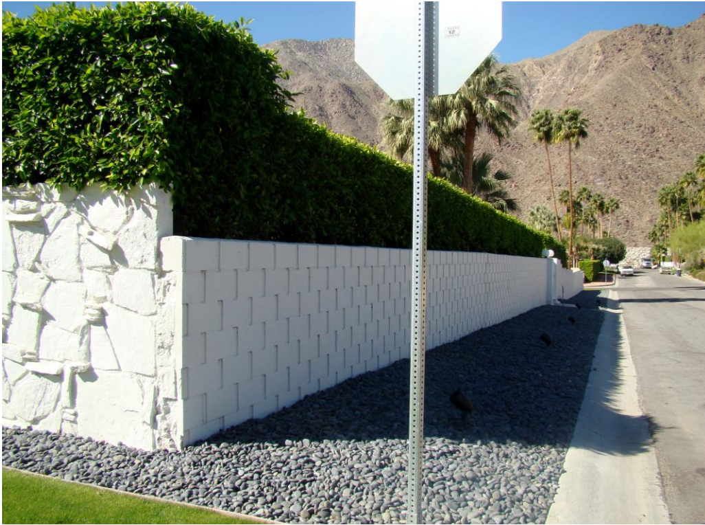
Wall of concrete block “Shadowal” on north edge of property. The concrete block wall surrounds much of the Morse Residence.
