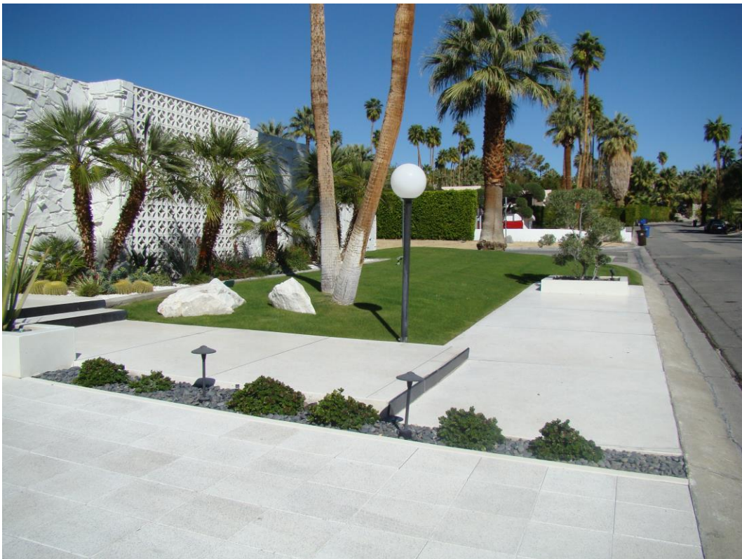
Terrazzo sidewalk and planters
